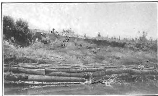
Timber toedam to prevent undercutting of levee.
