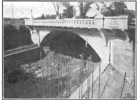
View showing the new abutments for widening the San Francisquito Creek 60-foot span arch bridge from present 30-foot to completed 76-foot roadway width.
