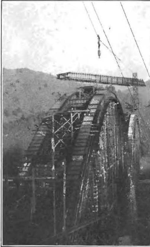
Placing a column form on Shasta Bridge No. 3. The reinforced arch has been partly poured.
