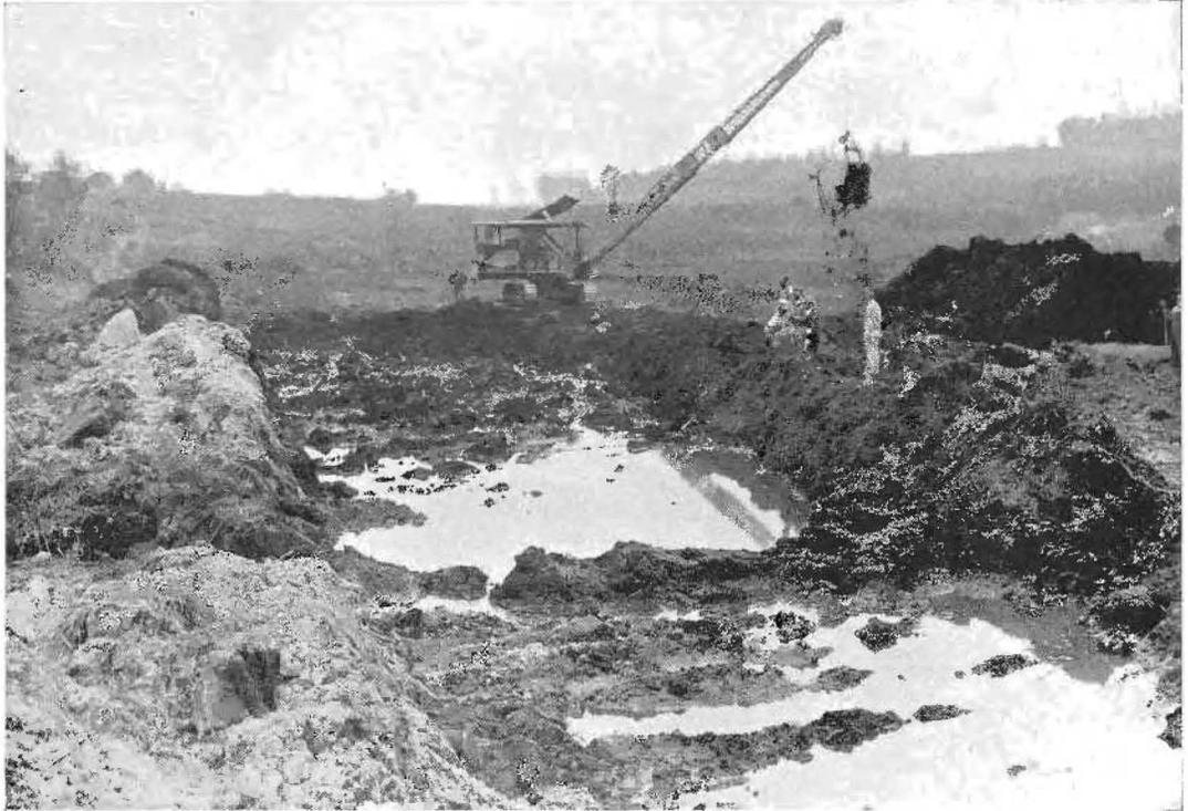
**TOUGH GOING** was encountered by the contractor on this portion of the San Juan grade realignment out of Salinas where the route lay through a mountain swamp. In the above picture is shown machinery working in a heavily watered peat bog. Seemed impossible to ever put a road there, but the bog was scooped out, filled, and today is part of the fine new highway cut-off to be opened early next summer.
