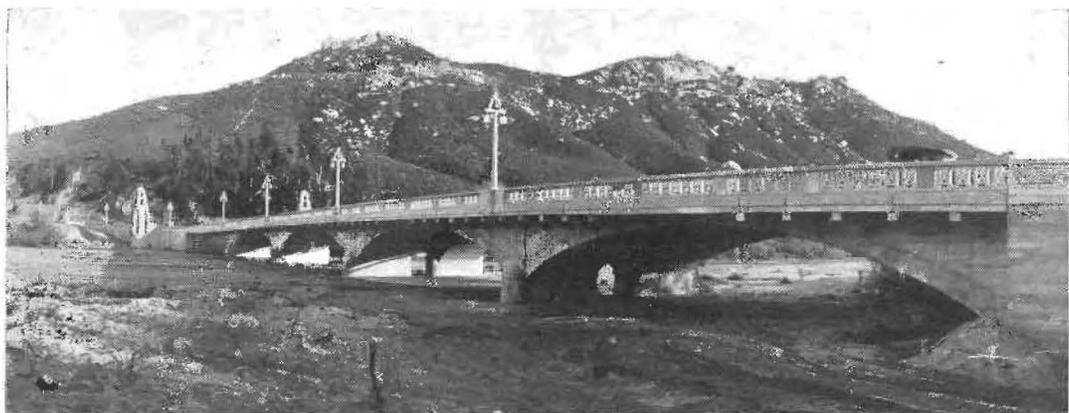
**RUBIDOUX BRIDGE**, at the foot of famous Mount Rubidoux, spans the Santa Ana River with five graceful concrete arches and carries the State highway over a 45-foot roadway to the western portal of the city of Riverside, beautiful Buena Vista Boulevard. The widening and rebuilding of both bridge and boulevard by State and city was celebrated with dedication ceremonies at which Governor Rolph and city officials officiated on March 29.
