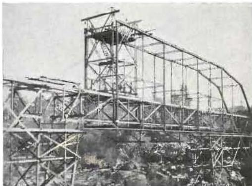
**ON ITS WAY**—Old Folsom span in process of being ingeniously picked to pieces and packed off to a new home on the Klamath River, 300 miles away.
