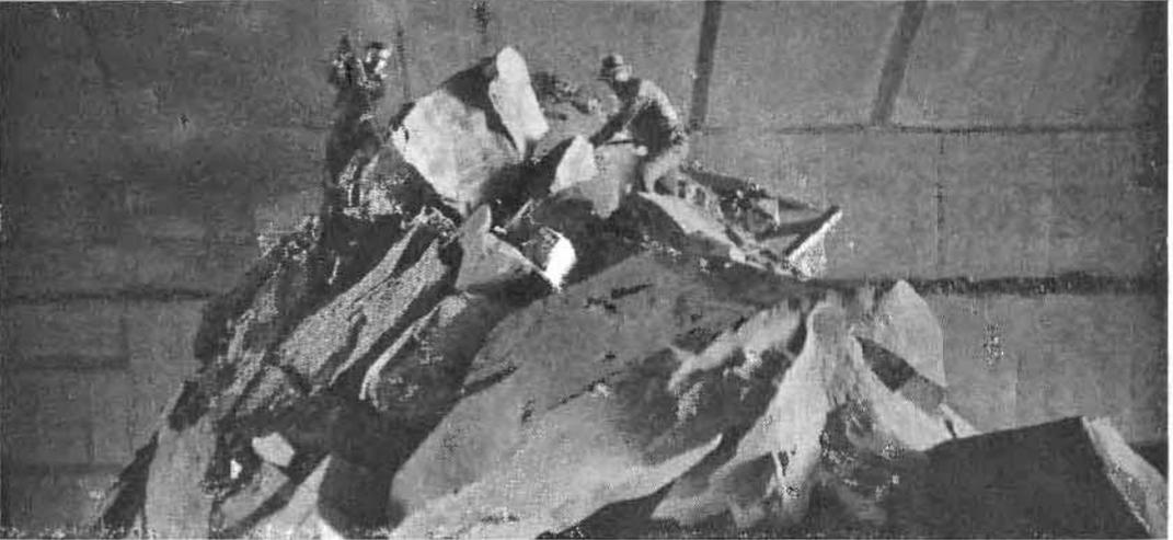
**REMOVING LAST OF CORE**—A horseshoe shaped excavation was made through the rock which was then concrete and steel lined before the inside or core of the tunnel was dug out.
