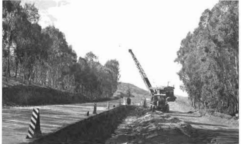
Drop-hammer operated from truck crane which compacted subgrade to depth 4 to 5 feet.
