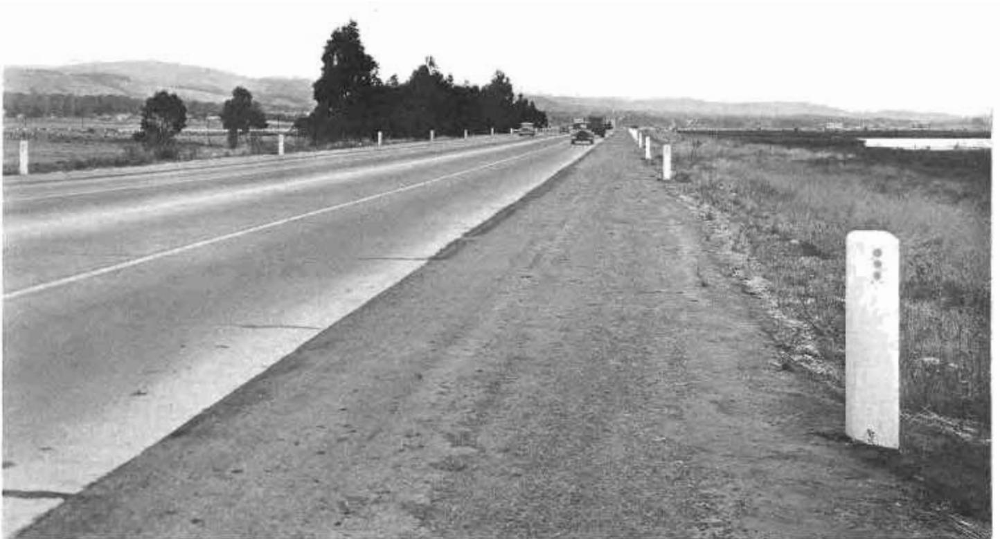
View of section of Bay Shore Highway between South San Francisco and Burlingame bordered by reflectorized sight posts being used in an experimental test of night delineation of roadsides. Each post bears three reflector units on two sides that are actuated by headlights of approaching cars.
