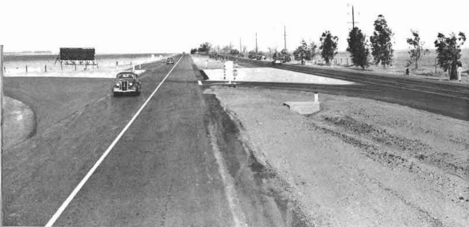
View of divided highway on U. S. 99 south of Bakersfield showing new lanes for southbound traffic on left separated from old highway by 26-foot strip. Islands for channelization of traffic mark the Maricopa-Taft intersection.
