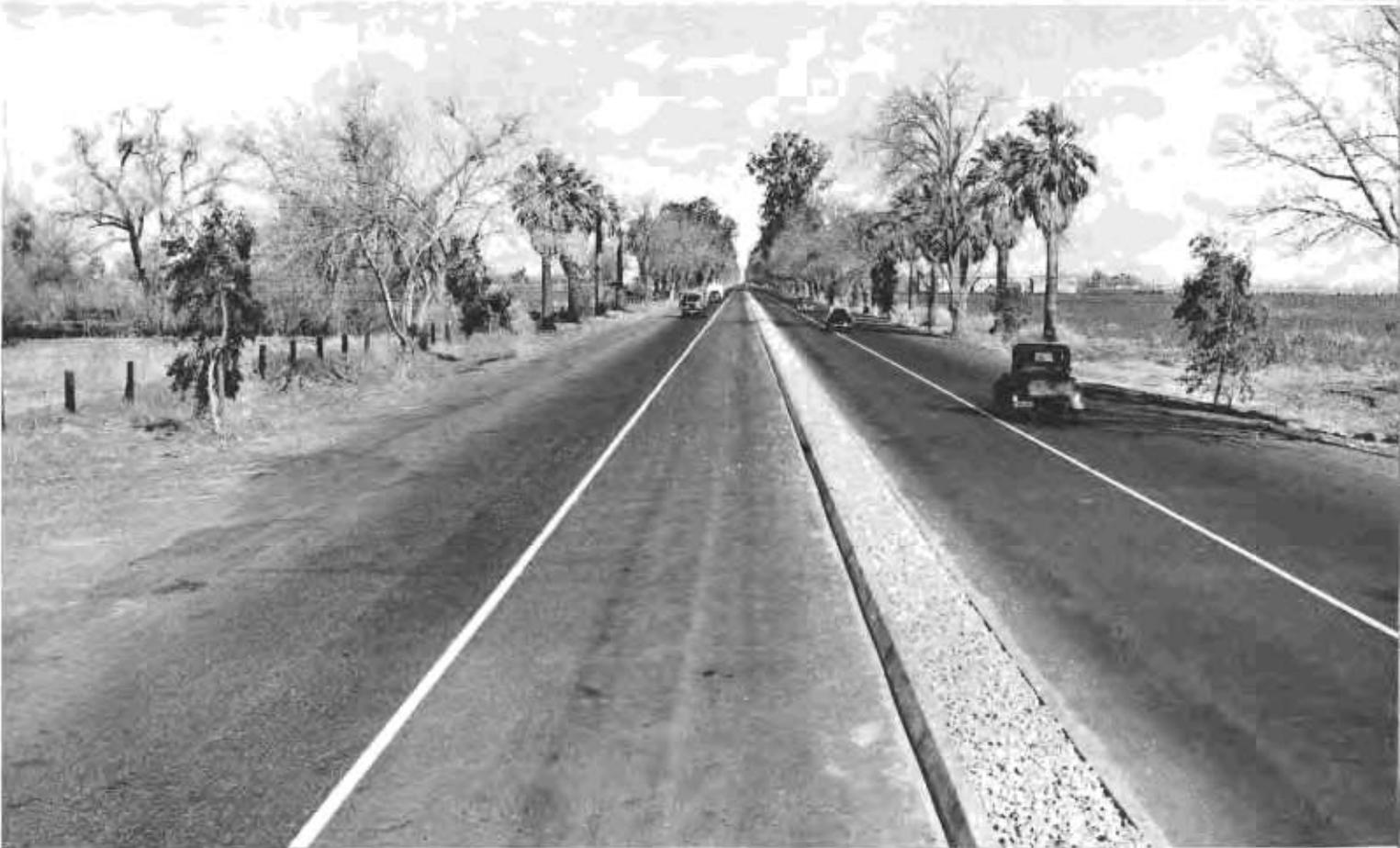
Two views of divided highway on U. S. 99 south of Bakersfield. The upper picture looking south shows the point where the curbed, crushed stone narrow dividing strip ends and wider tree covered separation divides the two lanes. In lower picture the dividing strip is located at center of old highway. Here the State owned wide, tree-bordered right of way that permitted extra traffic lanes to be built.
