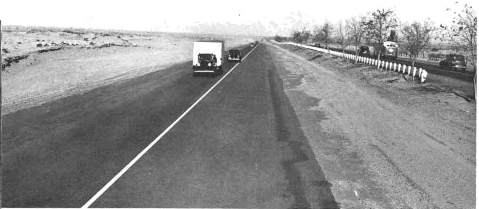
The new lanes for southbound traffic, at left, just added to the divided highway south of Bakersfield are shown at a point where they are separated at a different level from the old highway on right now reserved for northbound traffic.
