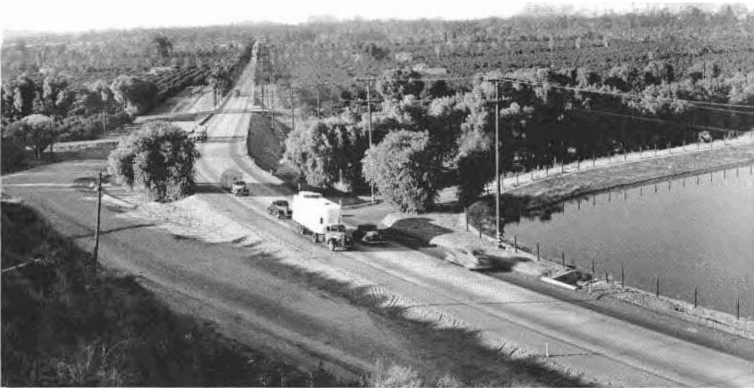
View of a section of the improved alignment on State Route 26 through Reservoir Canyon where the highway enters the orange grove area at the eastern entrance to the City of Redlands. The realignment eliminates steep and combined vertical and horizontal curves that presented dangerous conditions for traffic on the old highway. Part of the old routing may be seen at left.
