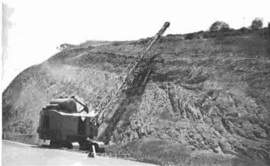
"Curry-comb" or spike-tooth slope grader on 75-foot boom attached to shovel.
