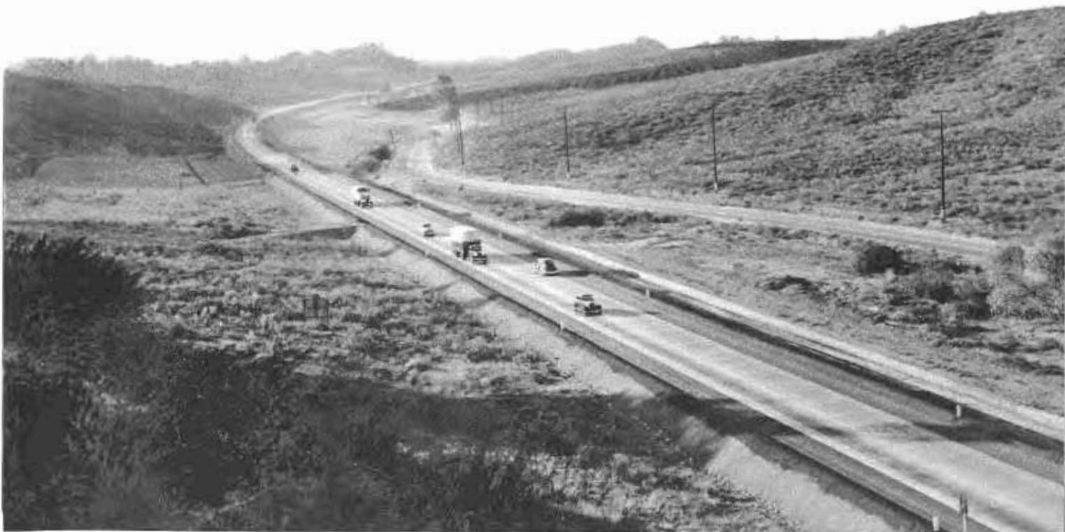
Another view of a part of the new State Highway alignment through the valley below Crystal Springs in Reservoir Canyon on the East approach to the City of Redlands. On the old traveled road, seen at the right of the new highway, numerous sharp, horizontal curves made dangerous driving conditions for the heavy traffic that this route carries.
