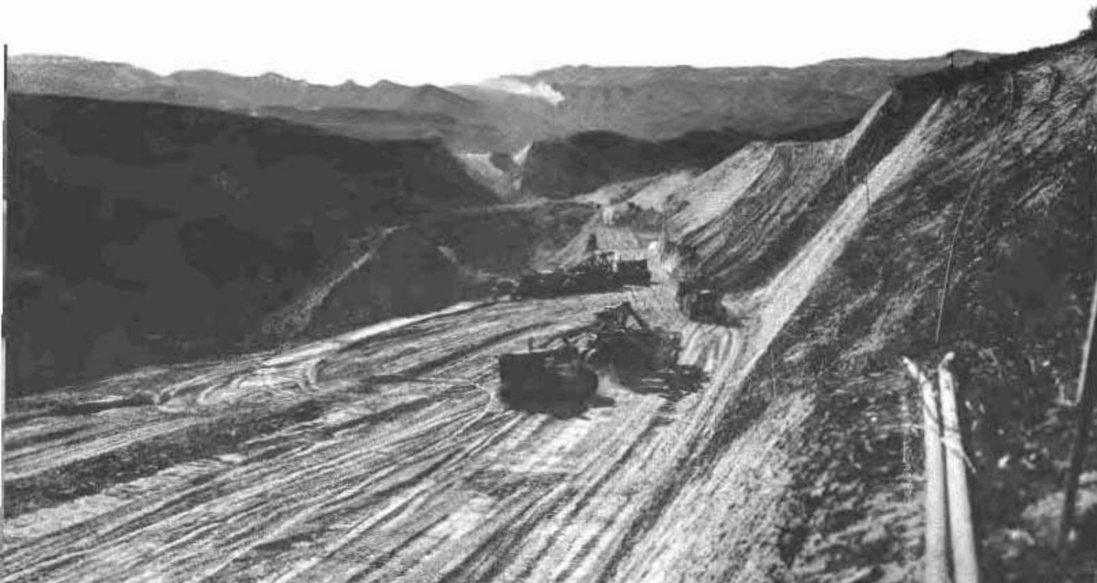
Rough grading operations on Mint Canyon Cut-off, with tractors pulling 25 and 28 cubic yard carryall scrapers.
