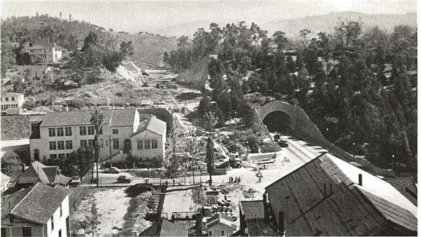
View of open cut under construction through Elysian Park in Los Angeles for southbound traffic extension of Arroyo Seco Freeway
