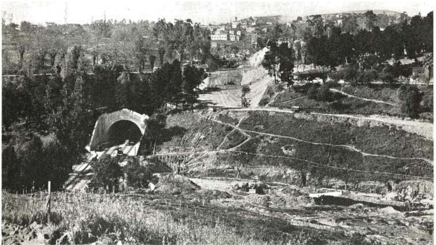
Open cut construction parallels existing Figueroa Street tunnels for northbound traffic seen at left. Large fill will be built in foreground
