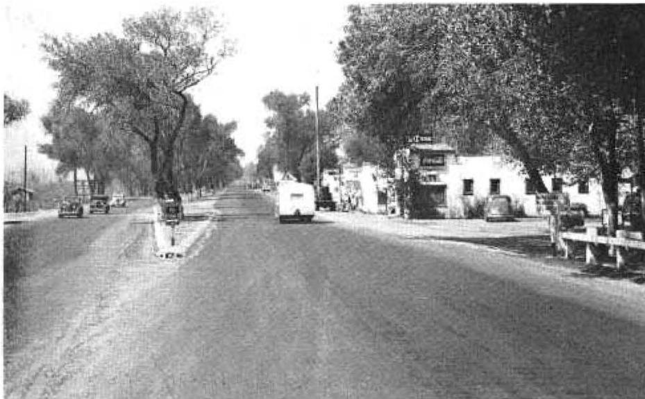
Flashing beacon marks dividing strip island which has cross-overs at intersections
