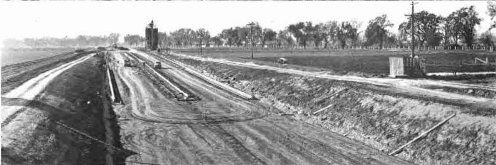
Progress of construction on the realignment of U. S. 40 between Davis and Dixon is shown in the above pictures. At top—Graded section approaching newly completed subway under tracks of Southern Pacific near Davis. Center—Building companion bridges across Putah Creek. At bottom—Grading operations for four traffic lanes and division strip
