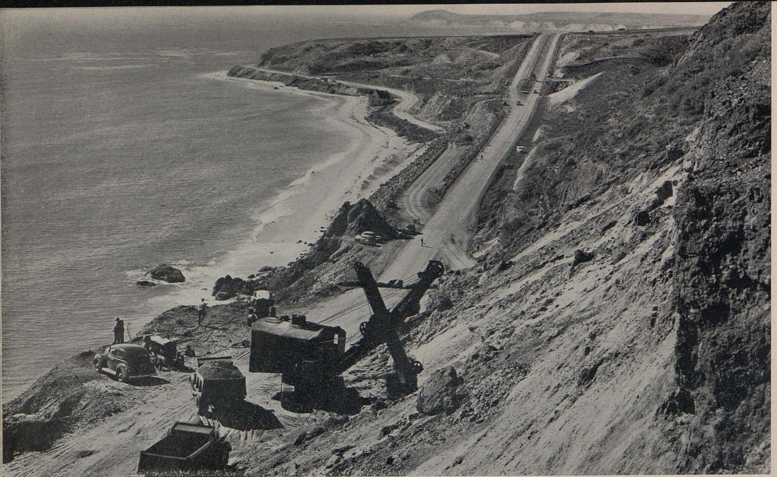
Two-yard power shovel removing 50,000 cubic yards deposit of beach sand on a bench 90 feet above coast highway
