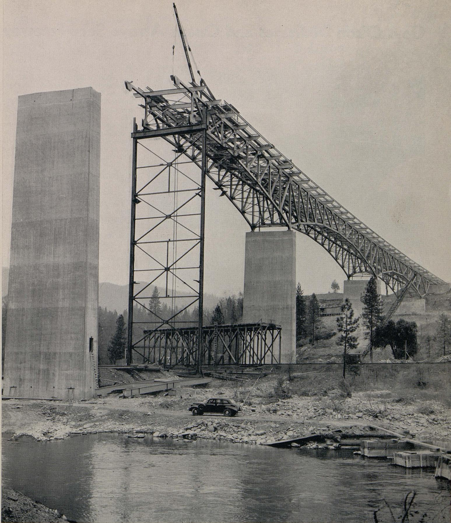
Highway bridge across Sacramento River at Antler on relocation of U. S. 99 made necessary by construction of Shasta dam. It is a steel deck truss structure 1330 feet long. The concrete deck will be 210 feet above the river
