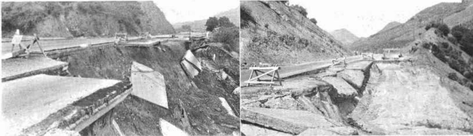
Views of slipout on Ridge Route Alternate, U. S. 99. Sketch shows method of correction
