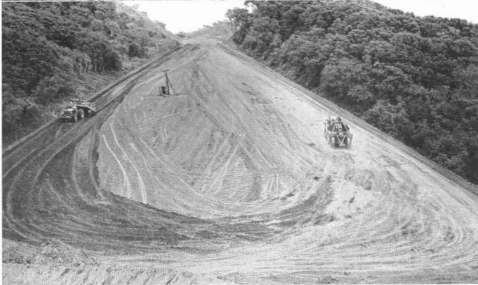
Construction on new Rob Roy-Watsonville Highway is proceeding rapidly. Upper—Truck loading with tractor pushing. In right foreground, Bulldozer in operation and in background, two Turnapulls hauling to fill. Lower—Huge fill being made
