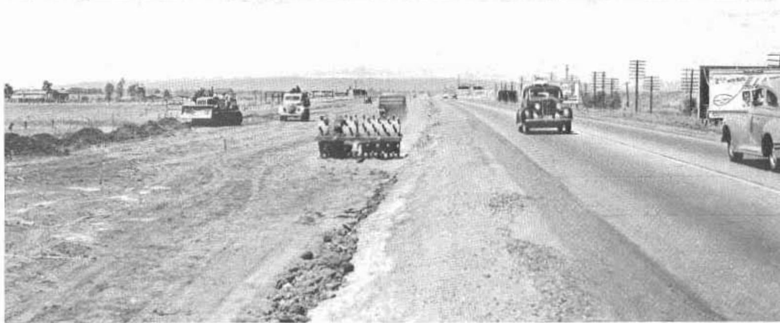
Views of realigned U. S. 40 between Davis and Dixon in Yolo County. Upper—Looking toward Yolo Causeway and Sacramento from point near State Nursery, showing resurfacing material windrowed in center of old highway. Center—Looking toward Davis; State Nursery on left. Bottom—Fill and widening operations for divided highway at point directly south of Yolo Causeway
