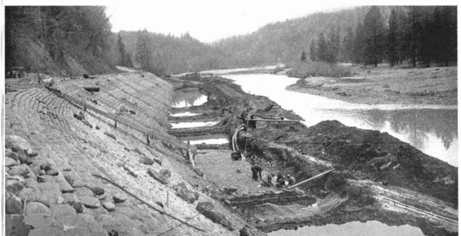
Workmen placing strip of wire and rock mattress in river bed at foot of riprap protected slope
