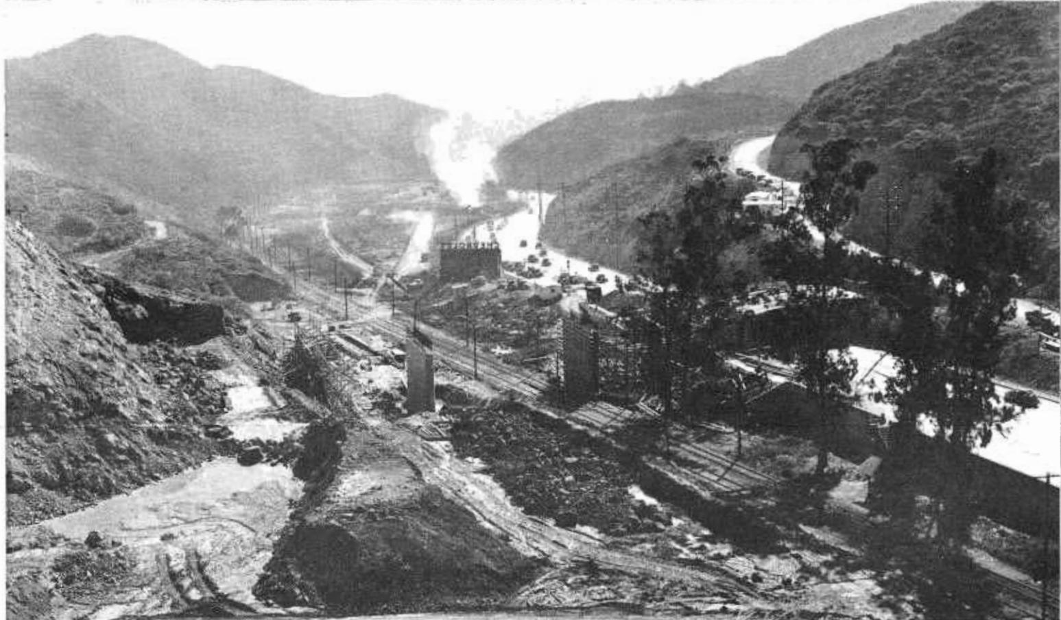
At top—General view of new Cahuenga Pass Freeway section looking south. Mulholland Drive overhead structure in foreground spans the old pass road retained as a service road on the right, the two 4-lane freeway roads, depressed railroad tracks and service road on the left. Lower picture shows scene during construction when railroad tracks were moved to a center position between freeway lanes
