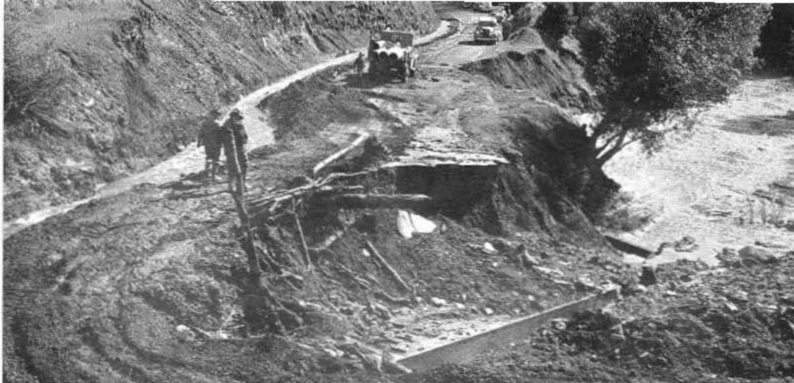
Washout on U. S. 299 West of Redding caused by February storms. Large sections of pavement were destroyed by undermining waters
