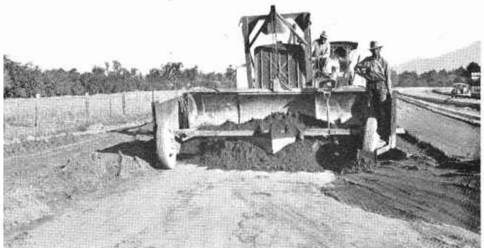
At top—Truck dumping cement stabilized mix in bulldozer spreader box. Below—Bulldozer equipped with forward steel wings attached to ends of blade and wheels spreading mixture approximately 14 inches deep on roadway
