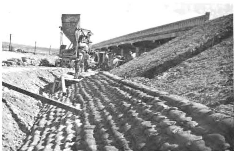
Sacked concrete riprap was placed at the ends of the bridge over San Gorgonio Wash to protect the adjoining embankments from storm damage
