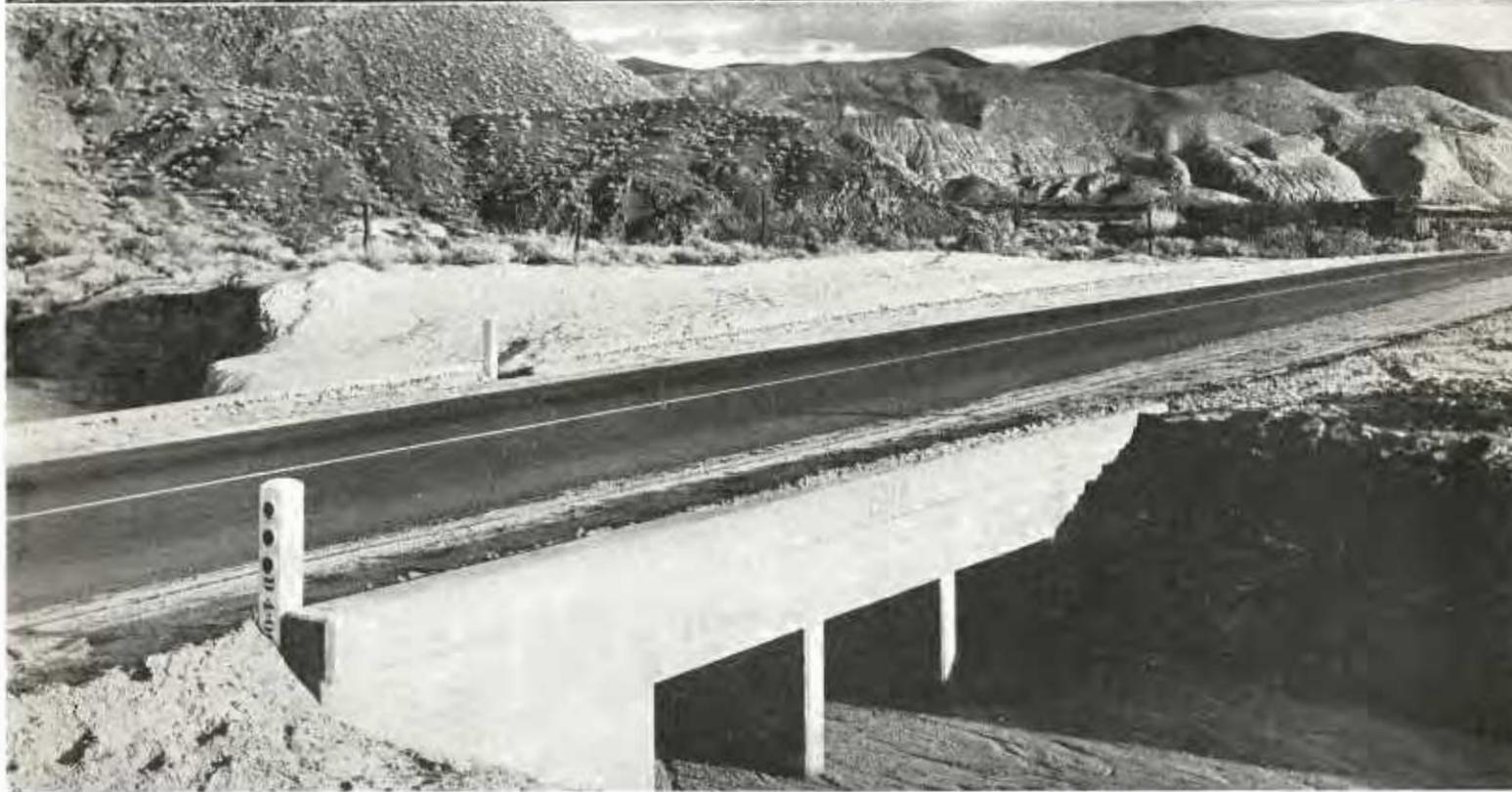
Views of sections of U. S. 6 Highway through Red Rock Canyon improved and made safer for traffic by elimination of dips. At top, dip replaced by fill and culvert. Center, a three pipe battery culvert and at bottom a triple box culvert
