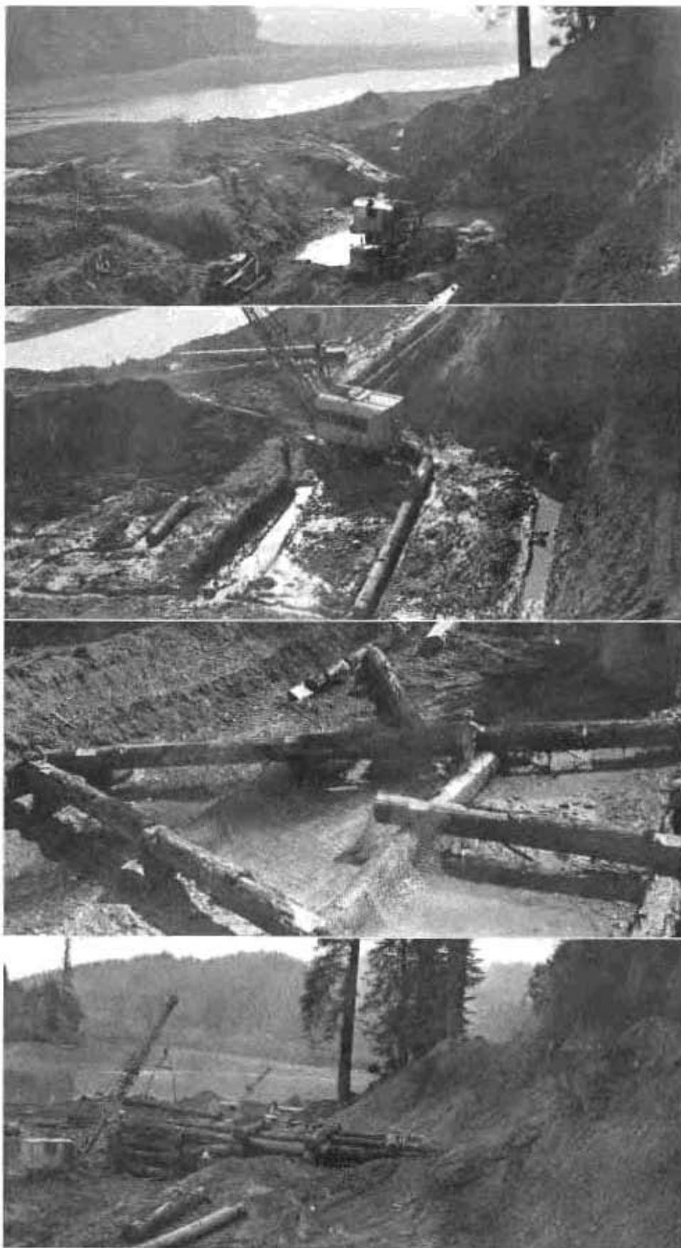
Pictures of deflector construction with 27-inch redwood logs from the foundation excavation to the completed structure filled with screened gravel of two-inch minimum size
