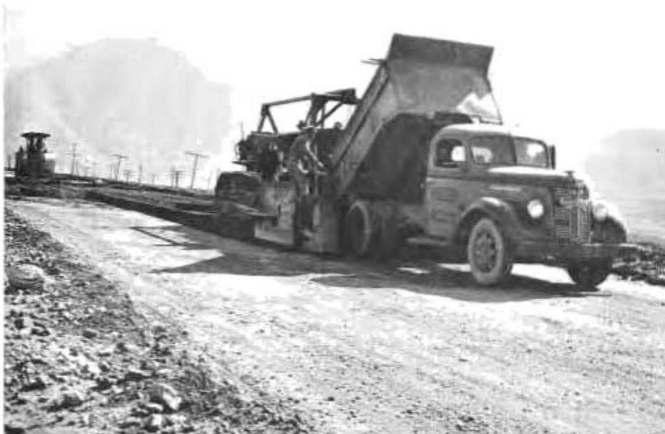
Spreading cement stabilized base. Note forward steel plate wing on bulldozer blade is mounted on wheel with screw jack adjustment
