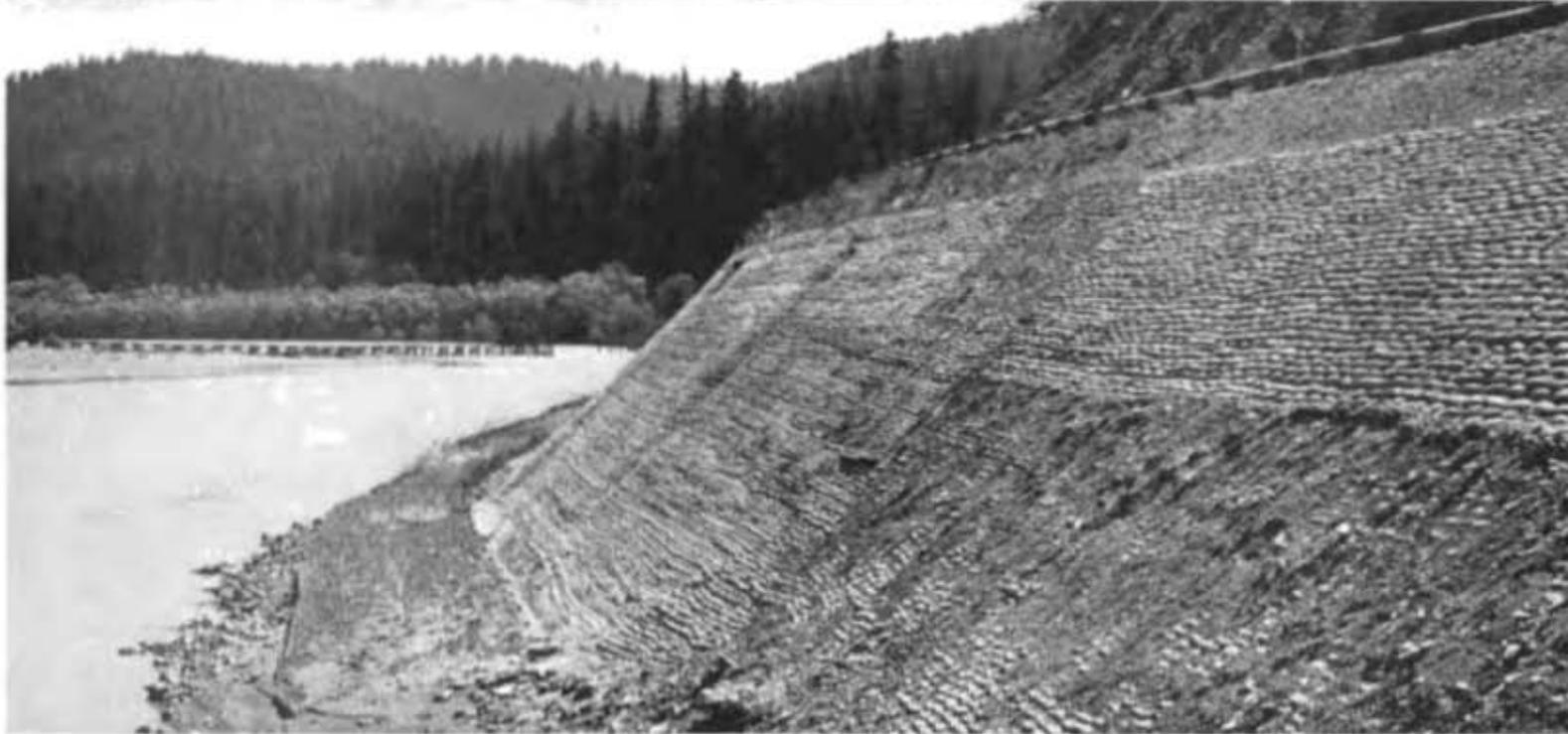
Triangular timber deflectors protecting banks and Redwood Tree groups shown above. At bottom riprap section that successfully withstood flood currents.
