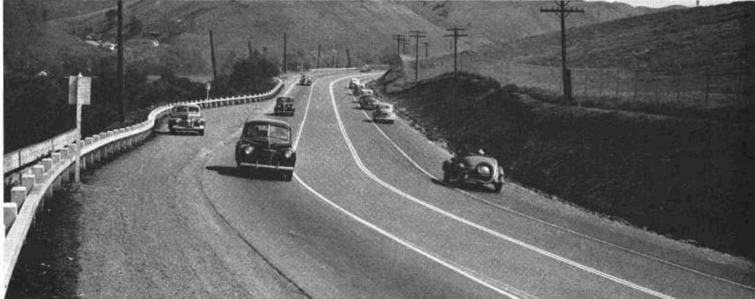
Three busy sections of U. S. 40 recently transformed from a three-lane to a four-lane highway
