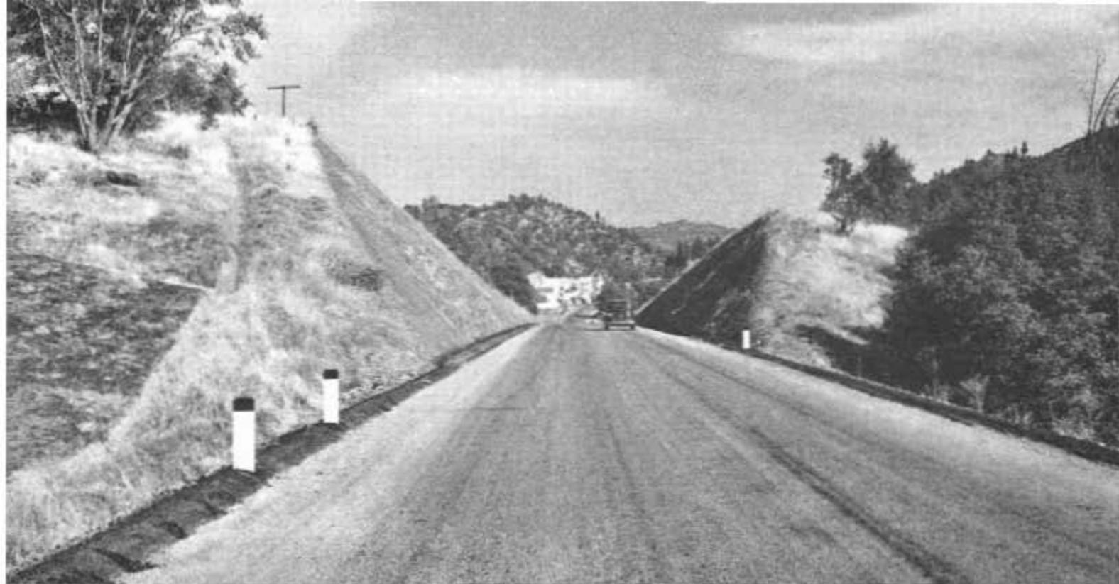
Road mix on gravel base surfaces a relocated section of State Route 18 in a mountainous area
