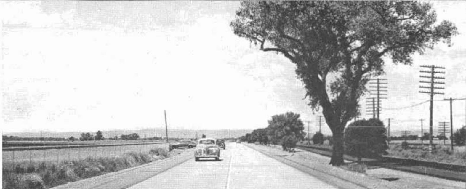
A 23-foot portland cement concrete pavement for one-way traffic on a recently completed divided highway section of U. S. 101
