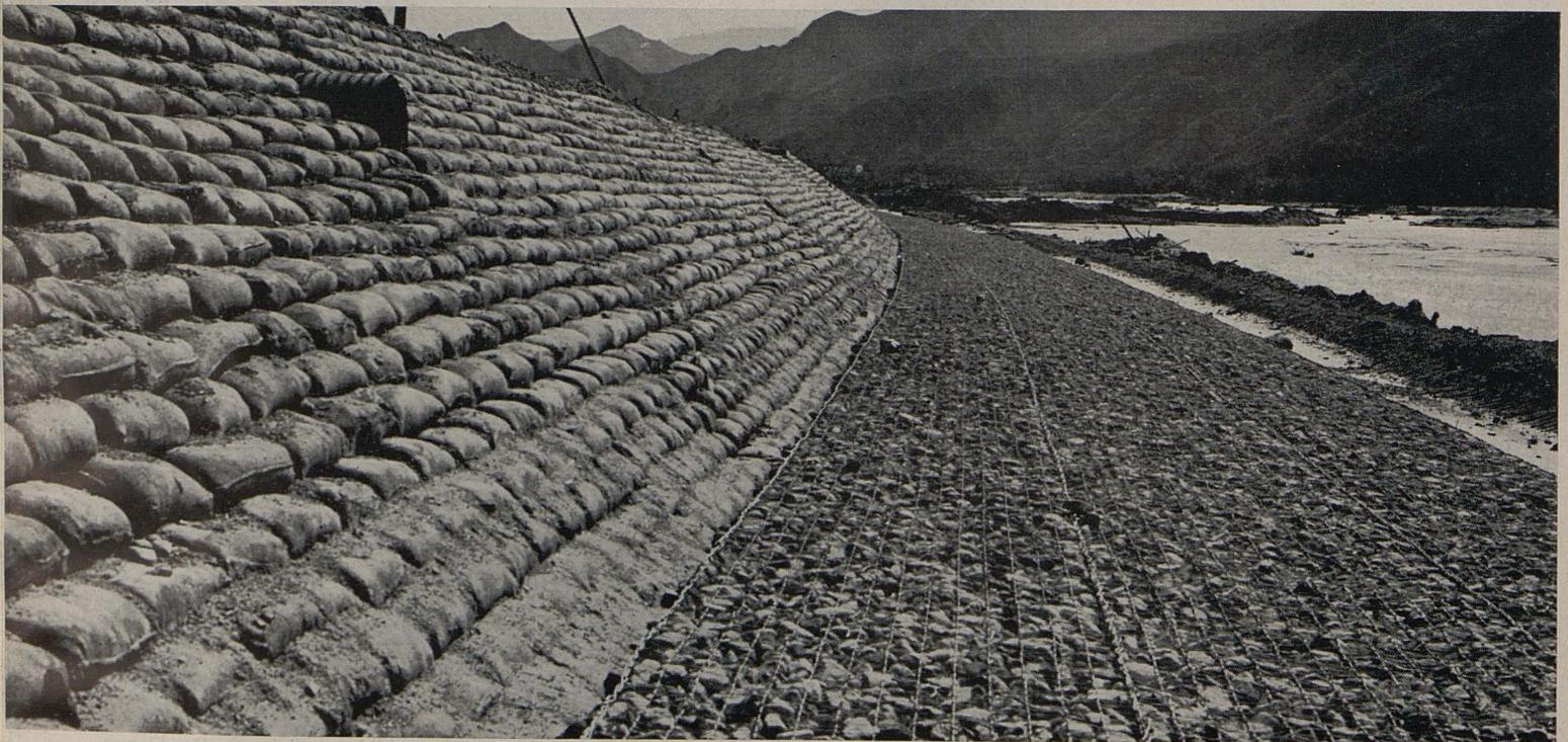
Sacked concrete riprap, 12 inches thick with rock and wire toe mattress, 8 inches thick and 14 feet 6 inches wide
