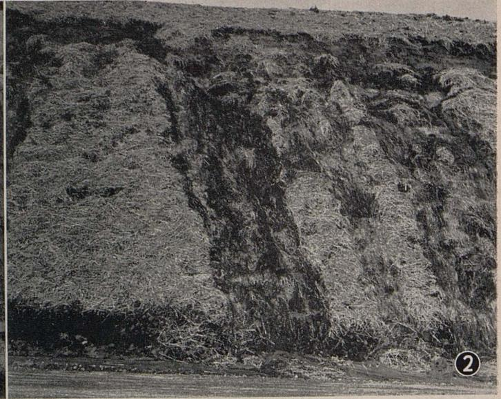
(1) Erosion gullies formed on a top soiled cut slope by 2.13 inches of rain. Note no intercepting drain ditches. (2) Result of 3 days rain, 3.95 inches in 24 hours, on newly treated slopes. Failure due to lack of bond of top soil to subsoil
