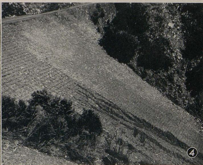
(3) Loss of top soil caused by first rain. No additional loss from subsequent rains has occurred. Soil is clay loam. (4) Fill slope protected by wattle method. On far half wattles were placed approximately 2 feet apart; on near half 4 feet apart. Note effects of erosion
