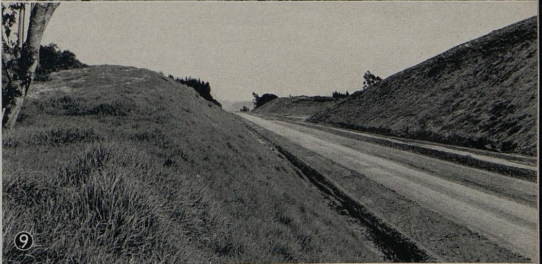
Typical erosion occurring on cut slopes during construction are shown in Nos. 7 and 8. On the same job and same soil  $1\frac{1}{2}$ :1 cut slopes are shown in No. 9 that were stabilized with top soil, rye grass and straw
