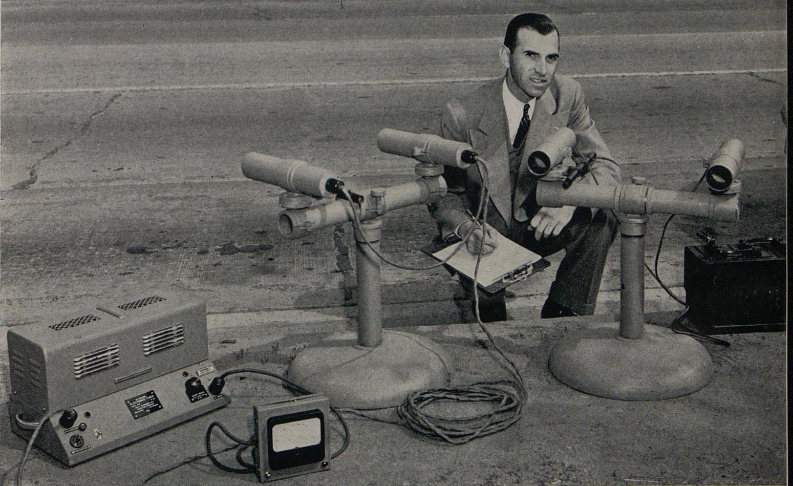
Views of new photo-electric roadside speed timer in action at top. Units of the apparatus are shown below with District Traffic Engineer W. M. Rieth who supervised its development
