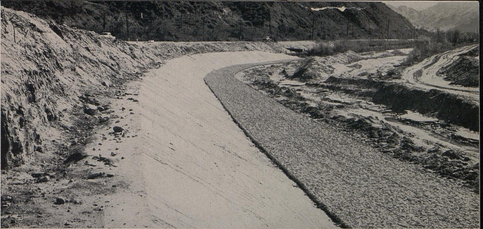
Portland cement concrete revetment on 1½:1 slope 10 inches thick with rock and wire mattress 14 feet 6 inches wide
