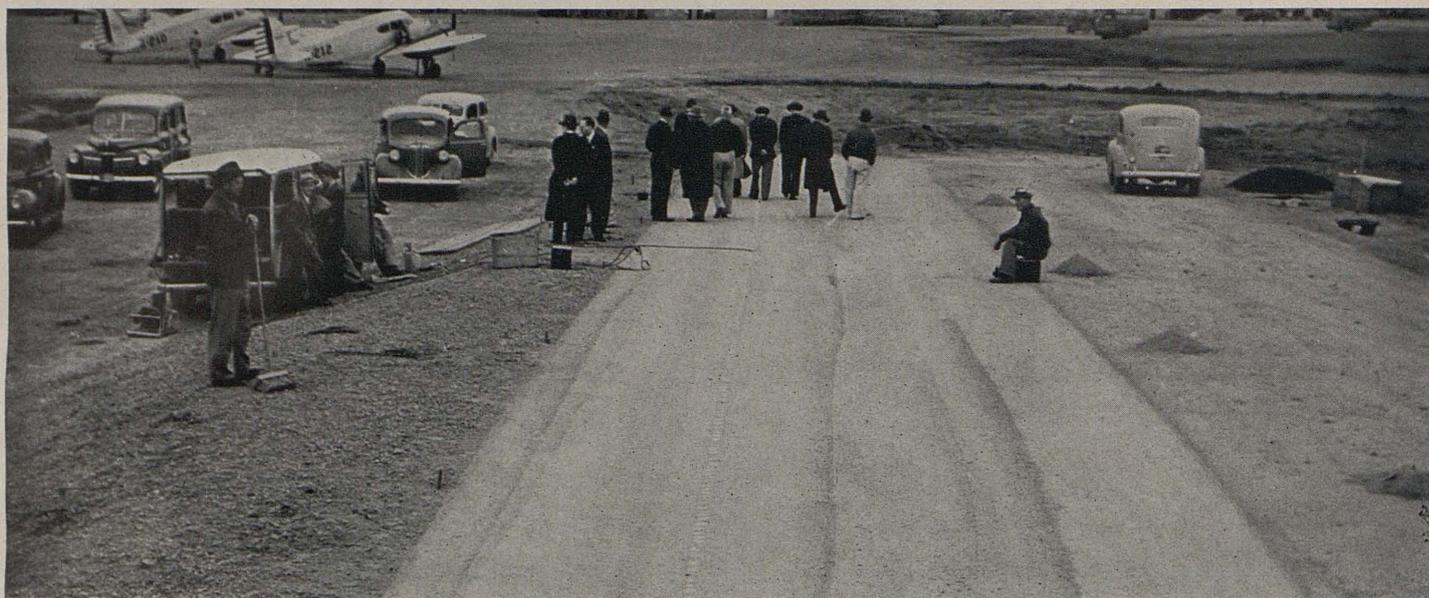
Army engineers inspect runway test pavement at Stockton field. Electric recording equipment for measuring subgrade pressure and pavement deflection under heavy wheel loads is mounted in station wagon at left
