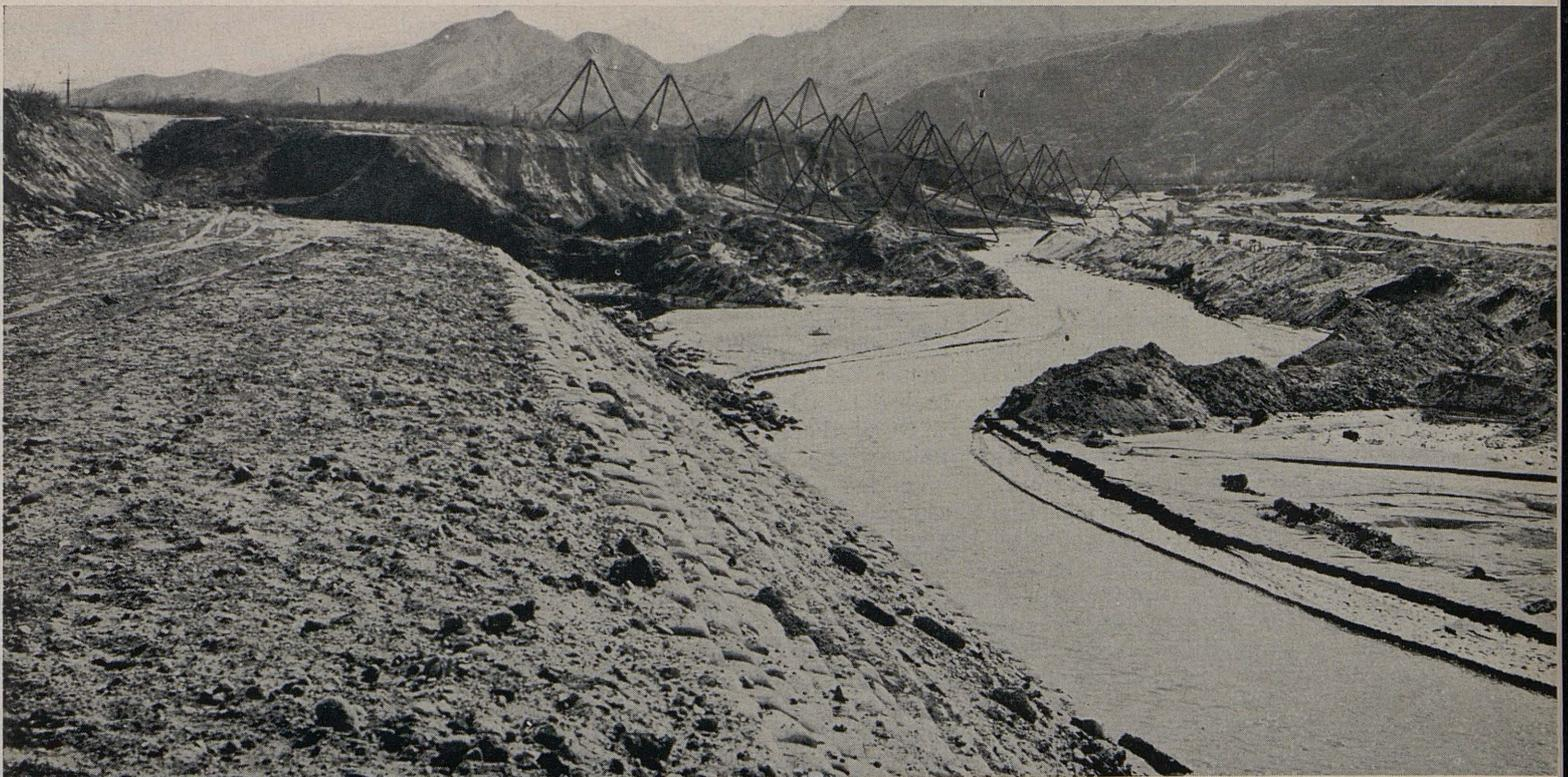
Thirty-foot steel rail tetrahedrons, shown in middle ground, and sacked concrete riprap installation in foreground
