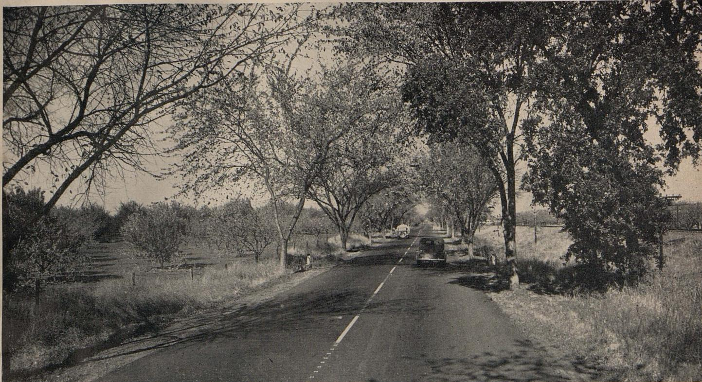
This photograph shows type of new surfacing on U. S. 99E north of Durham in Butte County
