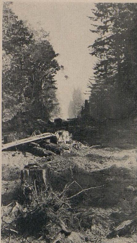
Grading a line change on north bank of Smith River, Del Norte, to by-pass a weak timber bridge
