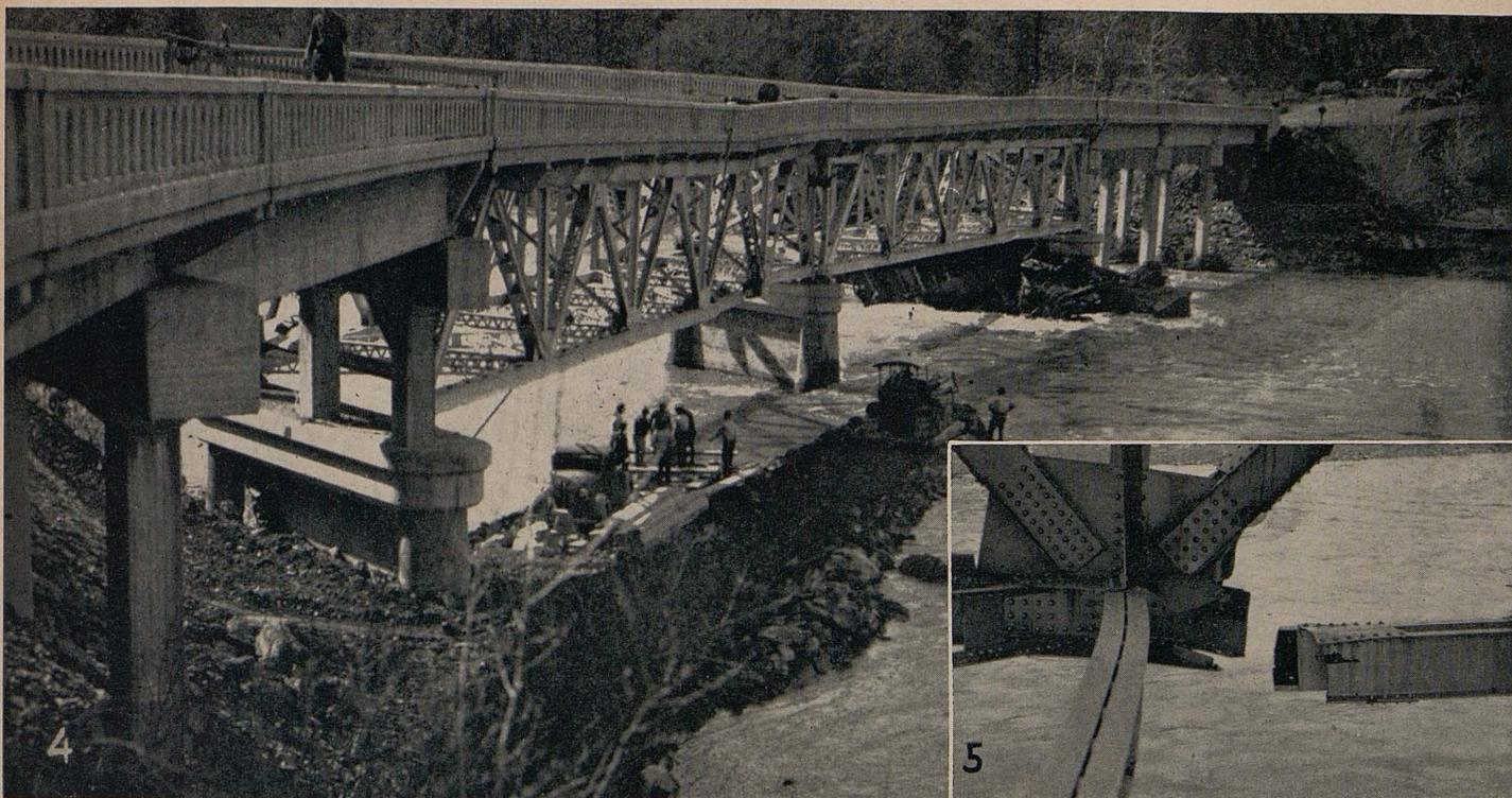
The damaged Trinity River Bridge with temporary repairs under way. Inset shows the severed lower chord
