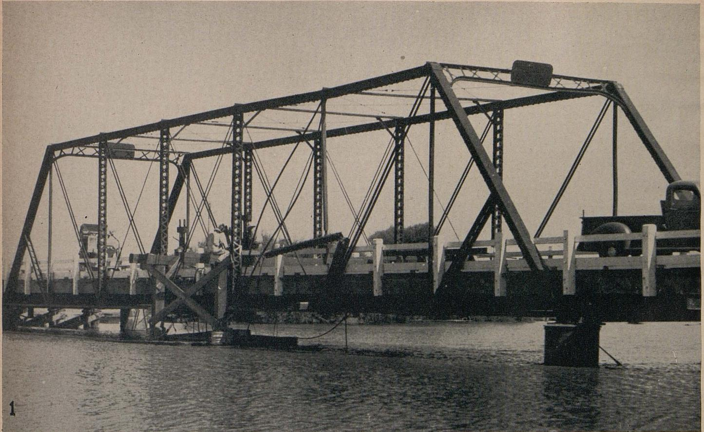
Repair of traffic damage at Kings Slough Bridge. Truss has been jacked back to grade through C. M. P. caissons and temporary supports placed under top chord. The broken vertical posts, bent almost double, shown in the center foreground
