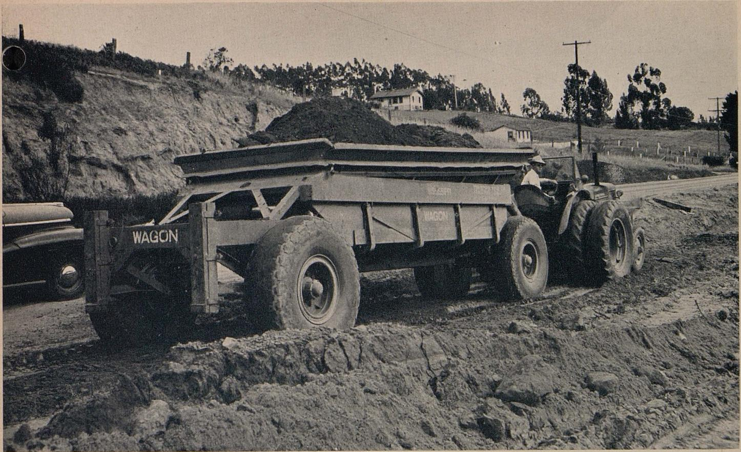
Mississippi wagon used to haul excavation materials involving hauls up to two miles
