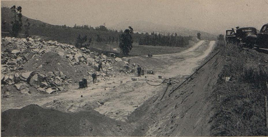
Drilling rock prior to excavating roadway cut near Mira Loma
