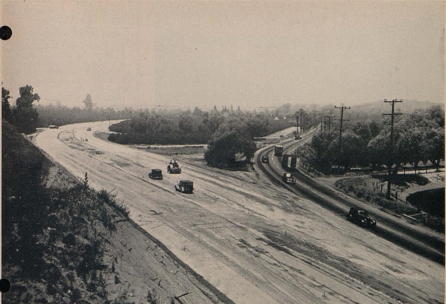
Redlands project showing old road on right and grading for new 4-lane highway construction on left
