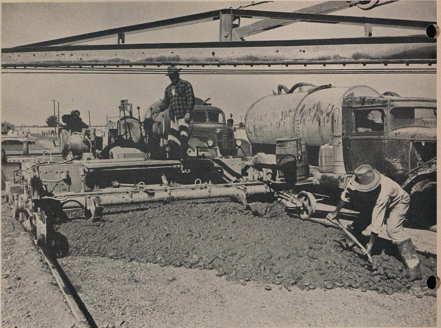
Vibrator spreader attached to tamping and kneading machine. Operator is backing up header where key is attached
