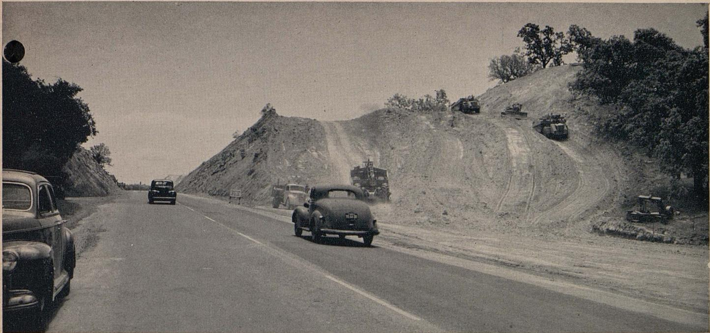
Woolridge Terra-Cobra scrapers excavating cut. The relation of the present road to the new construction is shown
