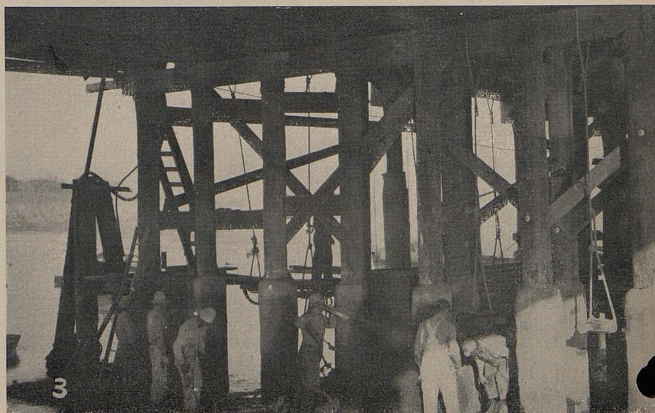
ments were completed. To stiffen the pile bents supporting the bulkhead, an foot "gunite" diaphragm walls were built between groups of three or four piles in these bents.
