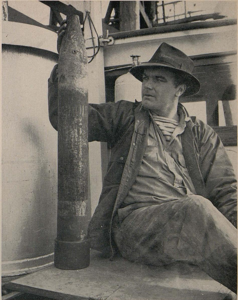
Close-up of jet nozzle. Four-inch pipe reduced to two inches
