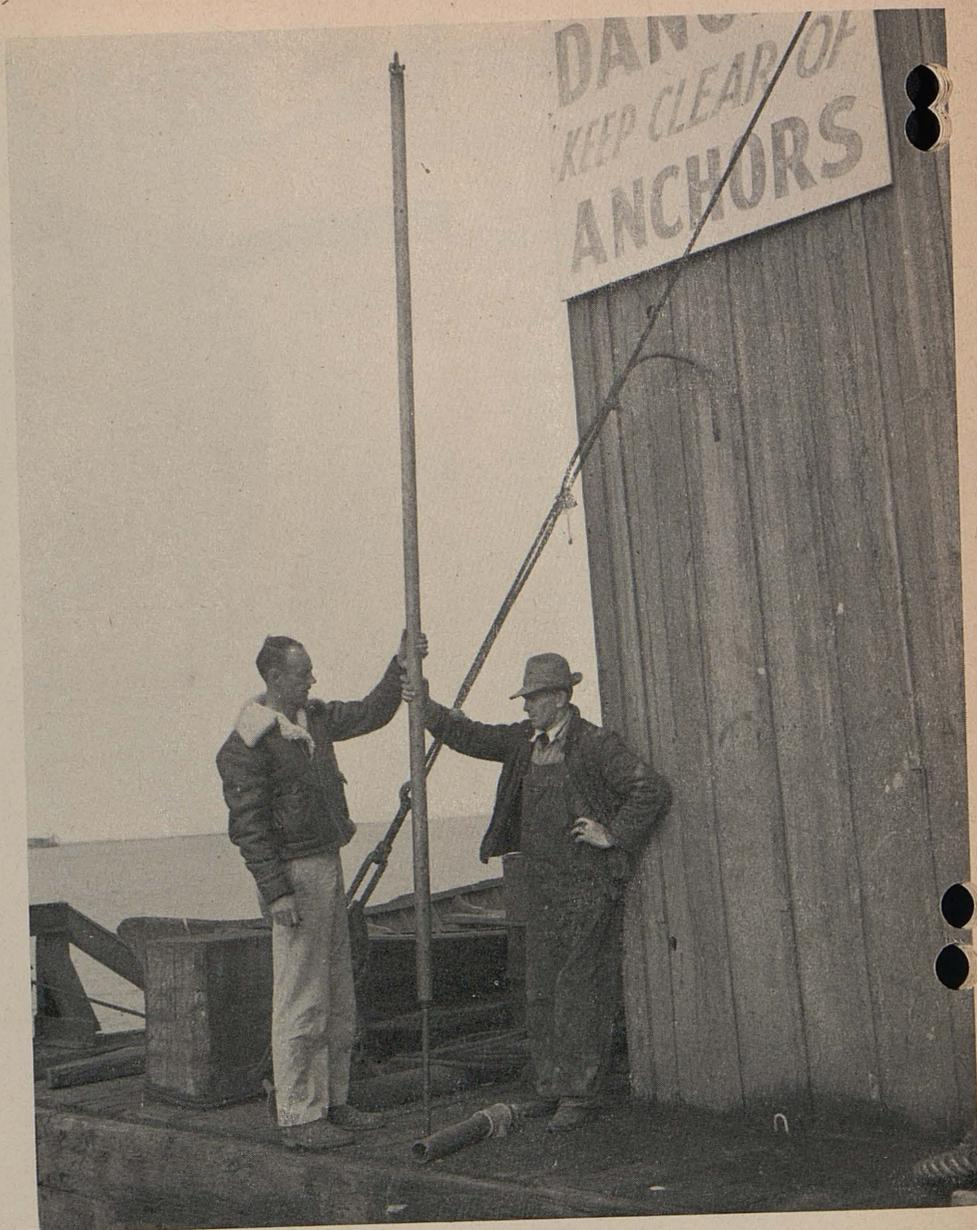
Sampler tube. This tube is weighted with lead to resist buoyancy
