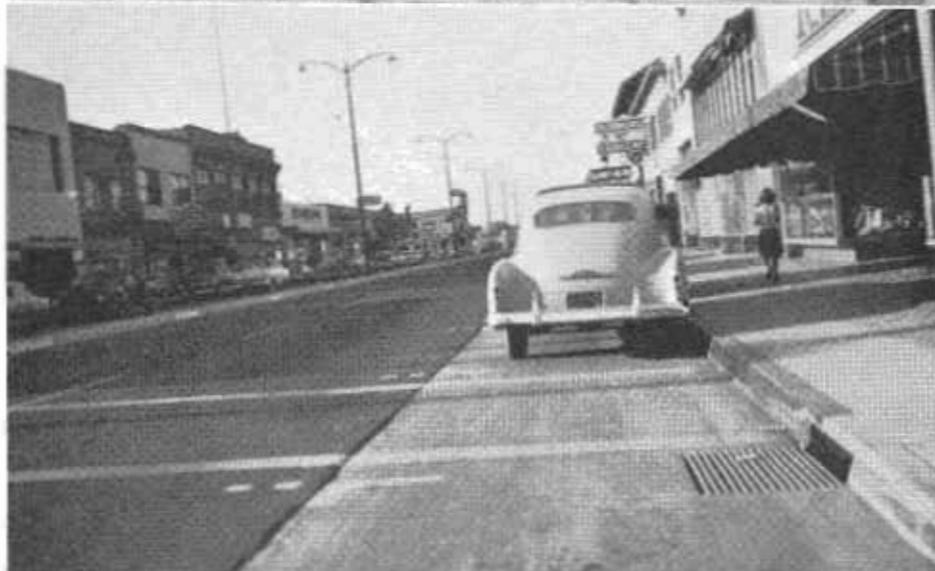
UPPER—Photo taken in 1951. LOWER—Photo taken in 1955. Both on Monterey Street showing the difference in typical parking conditions. The high crown and high curb shown in the earlier photo made it difficult to open car doors unless the car was parked some distance from curb, as shown in the photograph.
