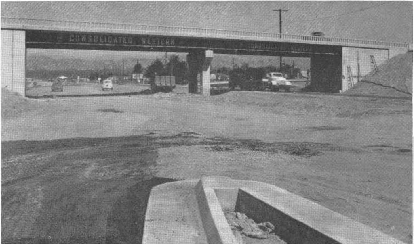
The mountains back of the City of Ventura are framed by the separation structure at the intersection with Saviers Road. Picture taken from southbound off-ramp prior to placement of untreated rock base and plant-mixed surfacing on southbound lanes. Pneumatic-tired compactor seen in center proved most effective in consolidating granular fills.
