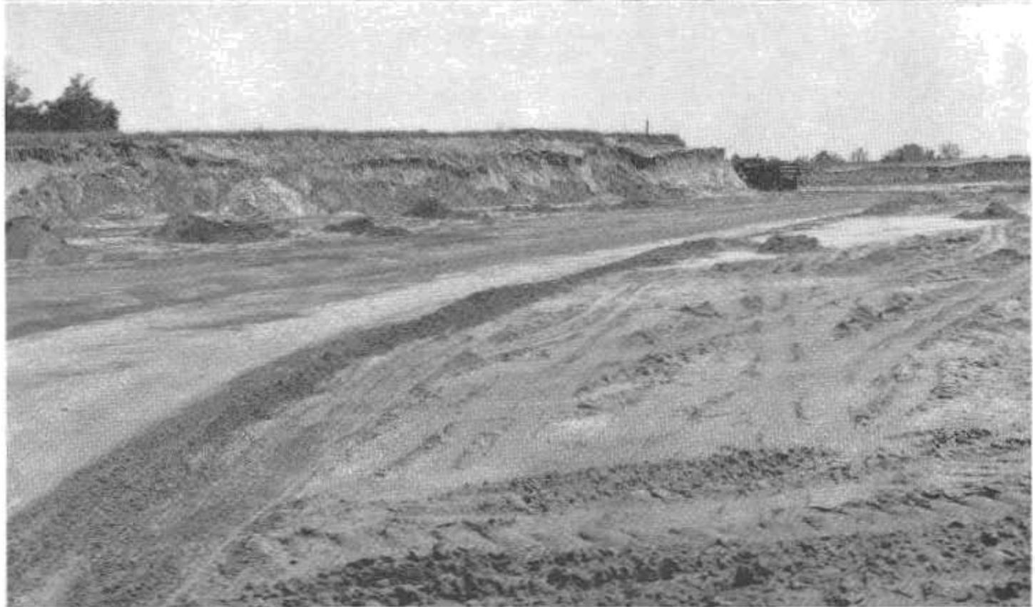
UPPER—Loading with a crawler-type belt loader pulled by a tractor. LOWER—Area of maximum cut showing high, previously unirrigable land being improved to an irrigable graded plane.
