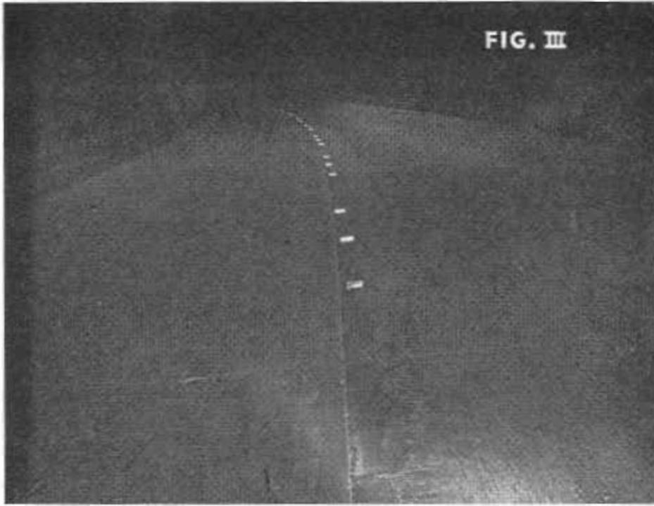
marker to the pavement may be speeded by the application of heat. Applying a butane torch to a small oven inverted over the marker for about three minutes and allowing the marker to remain in the heated oven for 15 minutes will generally induce a complete set so the marker will be capable of bearing traffic.
