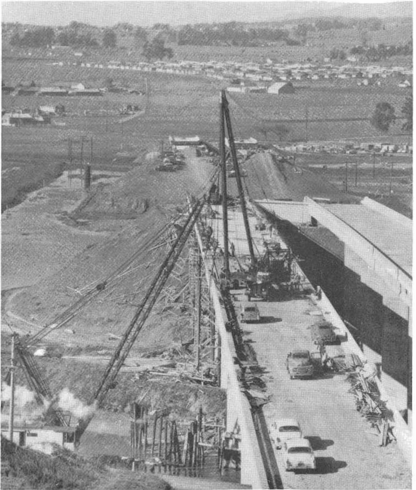
Barge crane and A-frame lifting final precast girder into place on northbound bridge over Petaluma Creek. Route 104 separation and overhead visible behind Petaluma Creek Bridge. Freeway right of way shown curving to left in background, looking north. This and other photos by Petaluma Argus-Courier.
