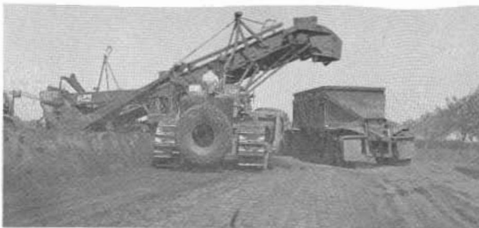
*Crawler-type belt loader pulled by a tractor required push equipment in deeper cuts*
