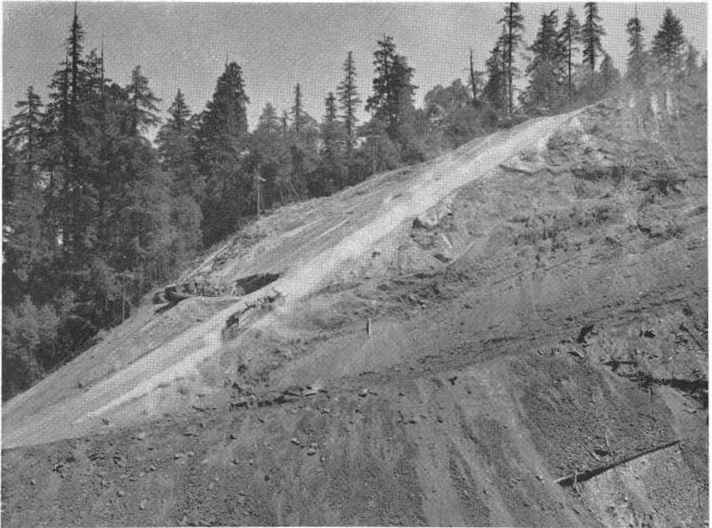
Equipment at work on the Big Cut. Steepness of the slope made it necessary to draw equipment to the top by the use of steel cable and winches.
