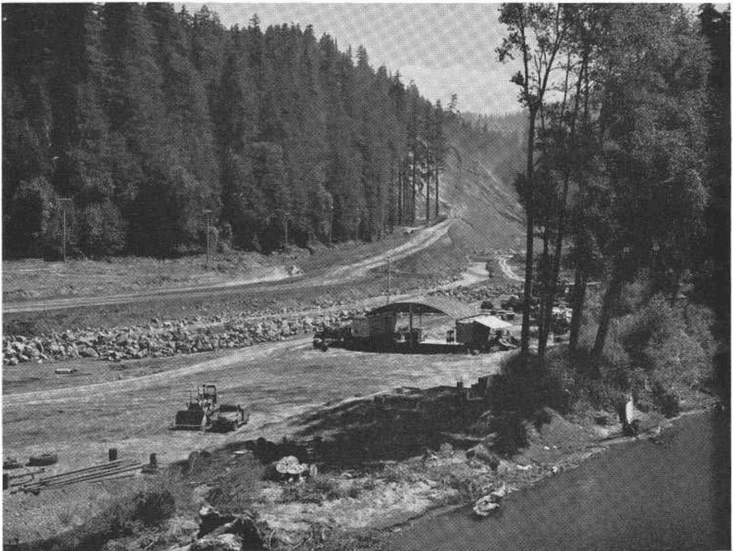
The South Fork of the Eel River shows none of the fury it unleashed in December, 1955, when it rose from elevation 110 feet to about 168 feet, overtopping existing US 101 in the right-hand portion of this picture. The projected cut failed to "catch" short of the top at elevation 650 feet.
