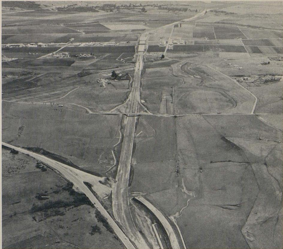
The first phase of construction on the Watsonville Bypass has been completed. For the next year the work will be allowed to stand while foundation materials settle; then the final phase of the work will be started. The view is southeast, toward Monterey County.
