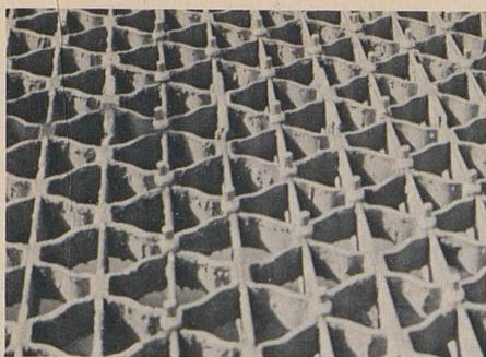
This photo shows the studs in place before being knocked off. The white collar around each one is an insulating ferrule used in the welding process. It breaks off with the stud.
