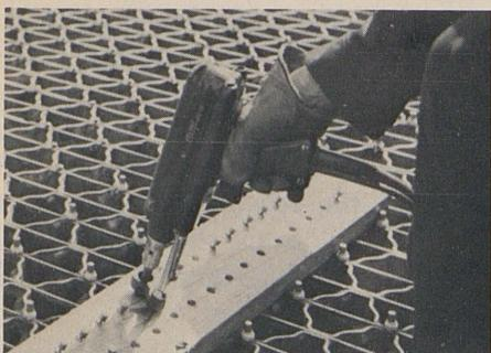
Studs were inserted in the gun from a holding board made by the crew to speed the operation.
