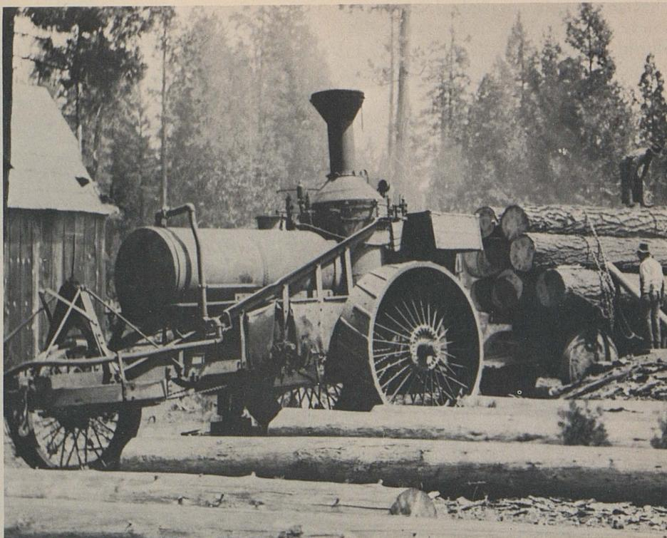
*A steam tractor used at the turn of the century to tow trailers transporting lumber from Shingletown to the railhead at Bella Vista.*
