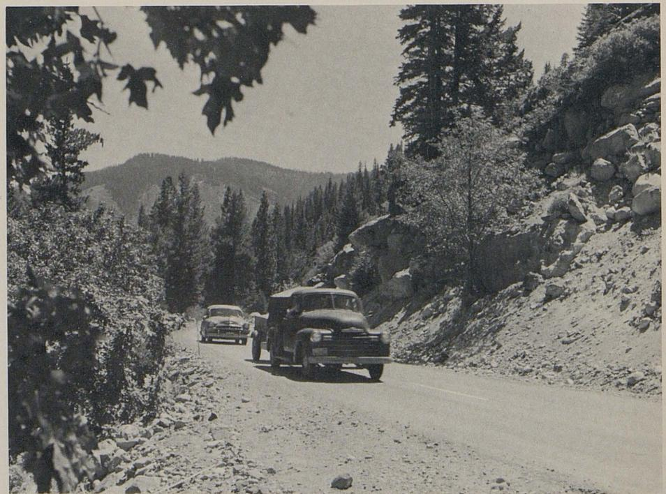
A typical section of the old highway before widening and improvement. Slope cuts (right) were through old glacial material of round, loosely packed rocks which presented a tough maintenance problem of constant sloughing and falling rock resulting from the freeze-thaw cycle in winter and spring.
