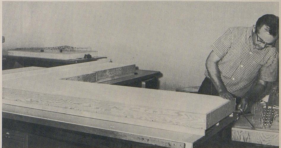
As a base for the models, blocks of styrofoam are combined as desired and framed with wood.
