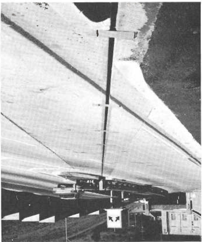
PHOTO ABOVE—A positive barrier, shown here in raised position, is designed to stop vehicles from crossing over into opposing traffic lanes. PHOTO RIGHT—Positive barrier in lowered position.
