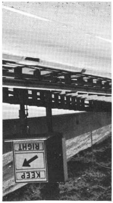
MESSAGE CHANGE. In the photo sequence above a button flips message prisms in a sign changing double arrows to single arrow and "keep right."
