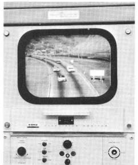
PHOTO TOP—Television camera set into the east portal face of the tunnel. Camera can be made to pan, tilt or zoom in on special area for closer look, all by remote control. LOWER PHOTO—A typical view of traffic as seen on one of the television monitors in the control room.
