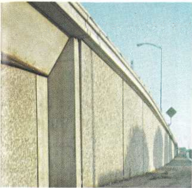
Above left: To add interest to long areas of retaining wall face, exposed aggregate panels were specified. The exposed pebbles are about 50 percent white, with the remainder ranging from light gray to black. (Fort Sutter Viaduct in Sacramento.) Above right: Here an interesting texture relieves what would have been a plain smooth face of concrete on these bridge piers. (The American River Bridge at Sacramento.)
