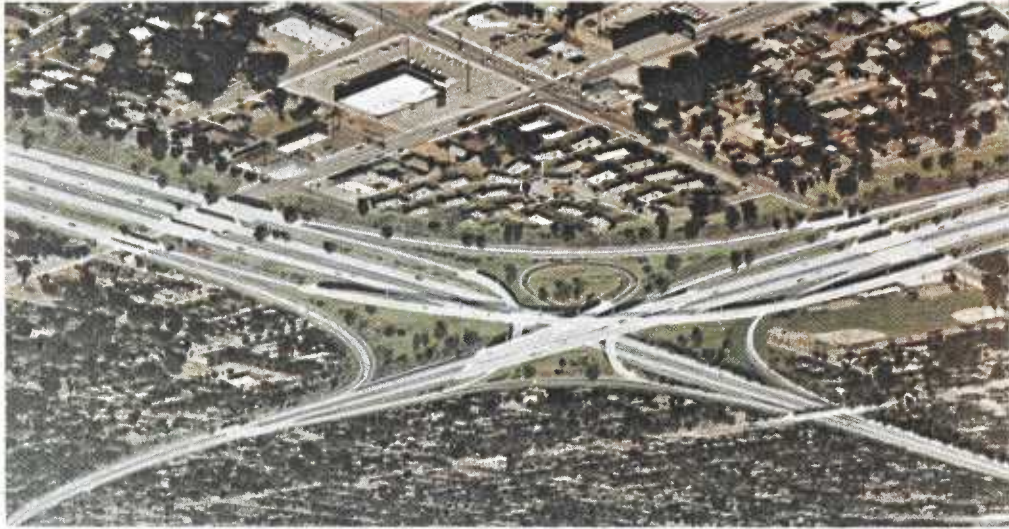
Above: Safety and traffic expedition are both served by the freeway which handles traffic at high speed which otherwise hopelessly clog the adjacent city streets. Note how landscaping separates freeway from residential area. Right: Route 99 through the City of Chico in Butte County. Bidwell Park is in the center of the picture. The viaduct through the park provides continuity for full enjoyment of this large park.
