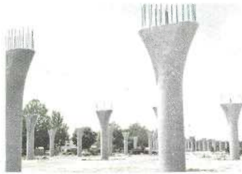
Above: Two examples of variations in design being used in current construction jobs in the Sacramento area. Since urban design involves the pedestrian's view as well as that of the motorist, new ideas such as these are being incorporated into structures to make them more pleasing in the city landscape.
