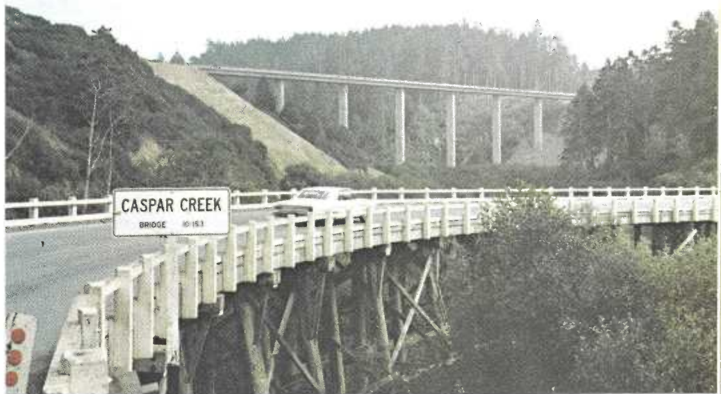
Above: The clean lines of the new concrete structure on its high, slim, rounded piers contrasts with the old sharply curved timber trestle which carried the traffic for past years (Caspar Creek Bridge on the Mendocino Coast.) Below: A high level, welded steel plate girder bridge which gracefully carries as many as 10 lanes of traffic over the Sacramento River. Although built on a huge scale, its lines reduce to a thin ribbon. (Pioneer Memorial Bridge in Sacramento.)
