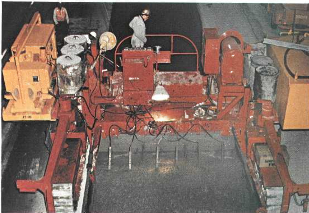
In foreground, finishers follow 12-foot slipform paver. Dump truck backs up to deposit batch. Empty truck en route to batch plant.
