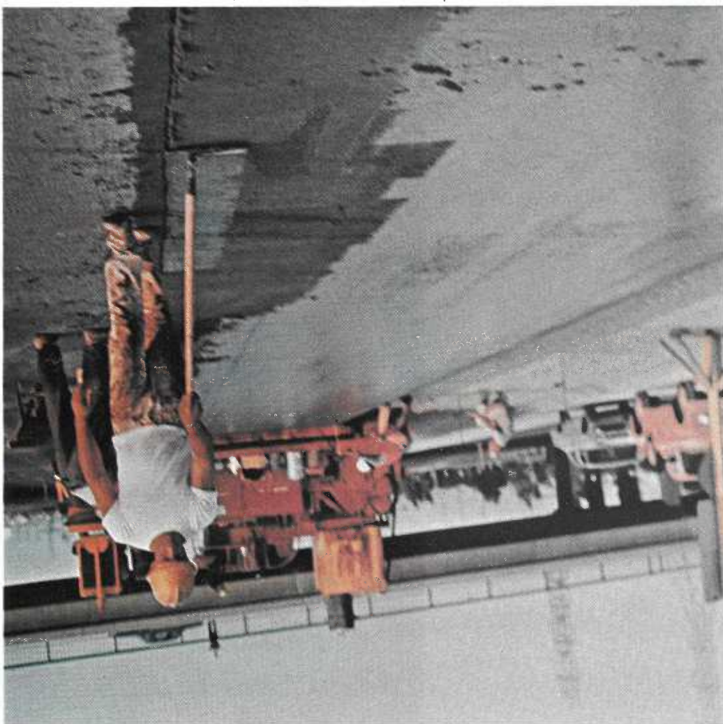
Finishing against existing pavement. Immediately behind paver, inspectors check concrete for grade.
