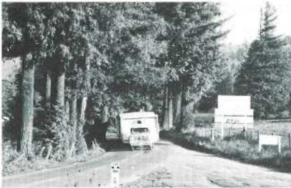
This narrow section and bad alignment on US 298 in the northwestern part of the state is typical of the hundreds of such deficiencies which still exist not only on secondary state routes, but on major federal and routes similar to US 298.
