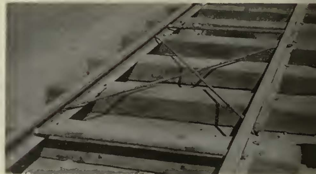
Rails are spiked on the outside to wood ties. The tierods run through pipe spreaders. Diagonal cross bracing is used to give rigidity to the section
