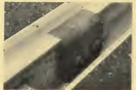
Repair of a broken rail made with a rail clip
