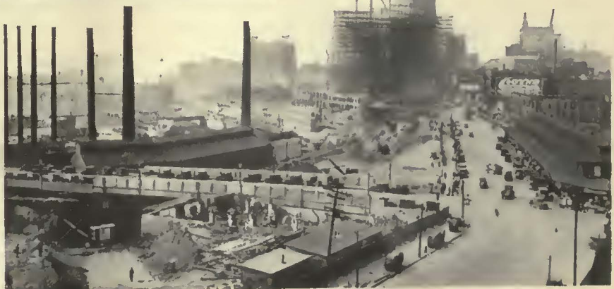
The station is approached from the west by a viaduct two-thirds of a mile long, extending completely over the Cuyahoga flats
