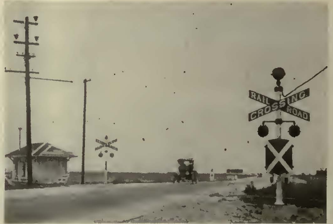
Nachod Highway Crossing Signal with flashing red lights and bell. An installation with two standards on the Galveston-Houston Interurban Railway.
