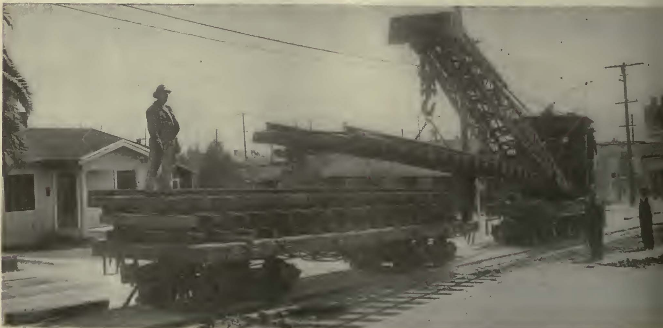
For transportation to some distant points, the sections of portable track are carried on a flat car
