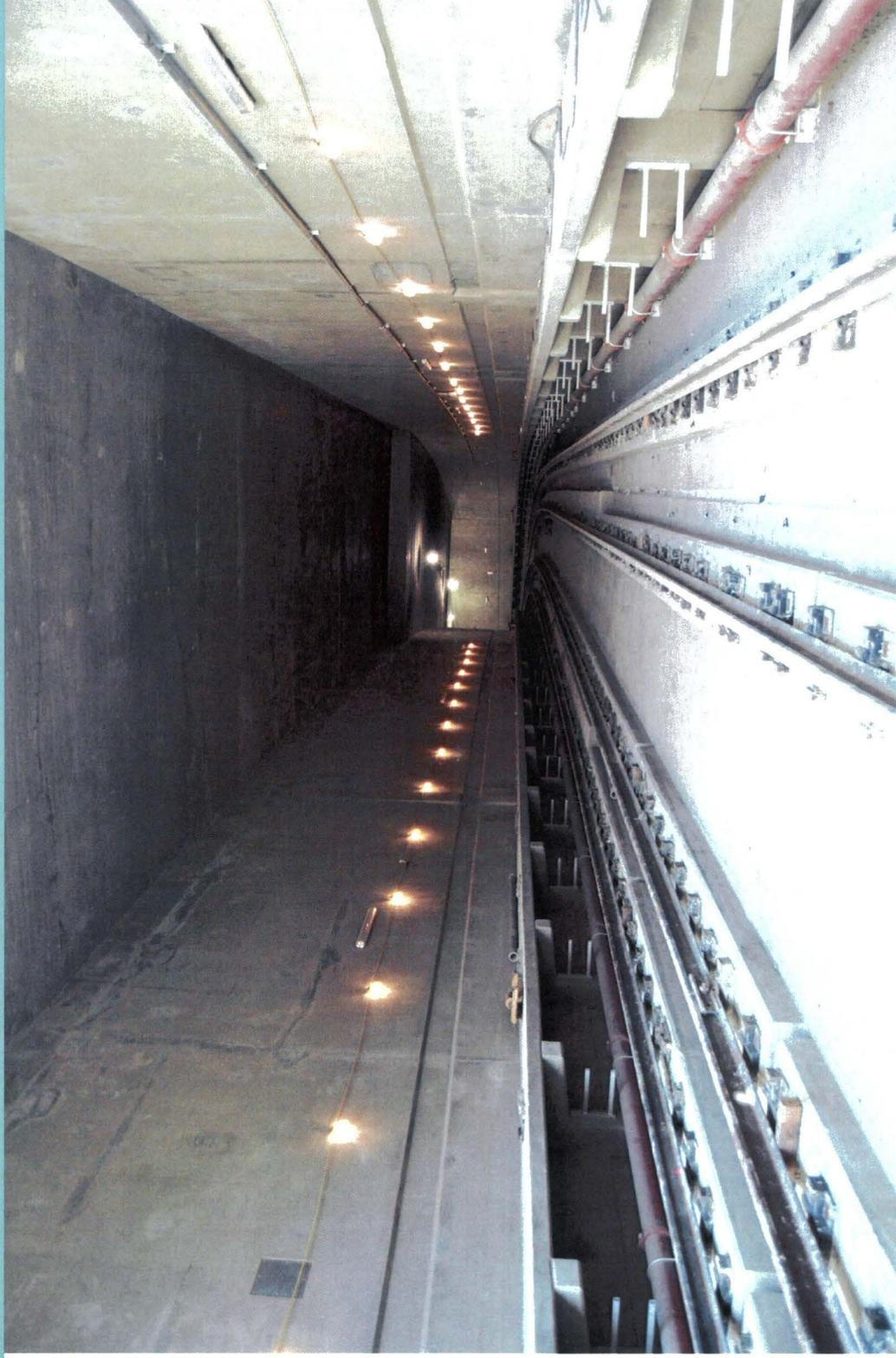
**Direct Fixation Trackwork in Trench Structure**
