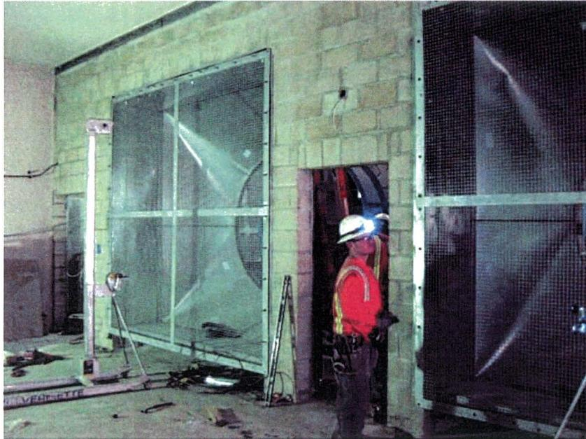
The underground ventilation system is being installed and inspected by the Metro Fire/Life Safety Committee.
