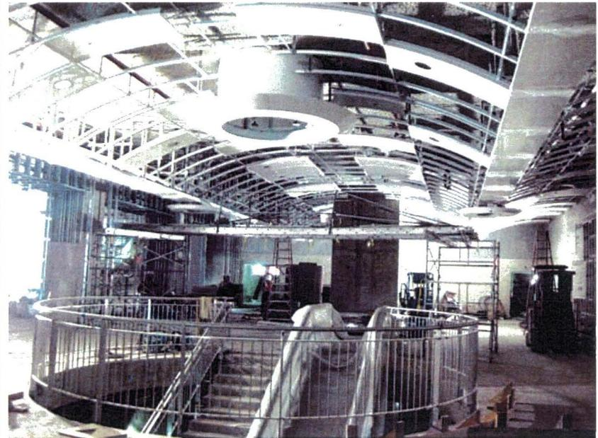
Architectural finishes, ceilings and ductwork for the ventilation system are being installed in the underground station.
