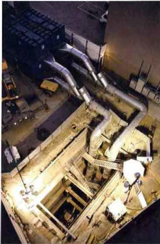
**Exploratory Shaft Contract C1034** - The temporary exploratory shaft was constructed to gather data related to soil conditions, gassy ground and ground water to assist in the geotechnical design of the Wilshire/Fairfax Station and tunnels. Risks associated with potential construction delays during the discovery and excavation of prehistoric fossils will be mitigated through planning of early construction activities.
