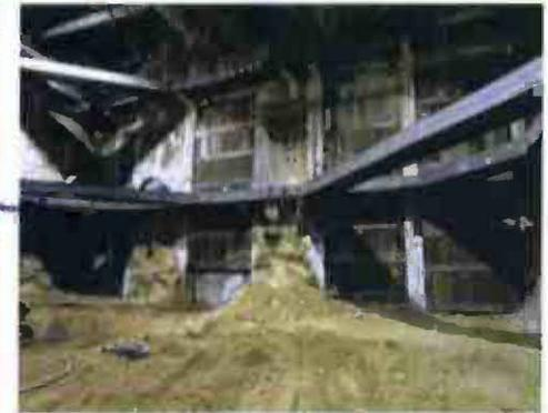
EXPOSITION STATION – Timber lagging operation at south headwall
