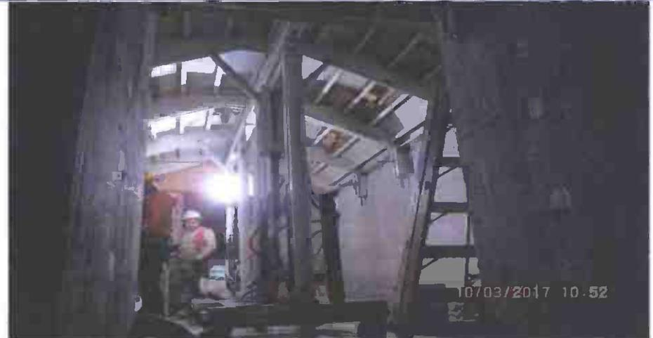
**TUNNELING – Erecting arch section formwork at CP-5**
