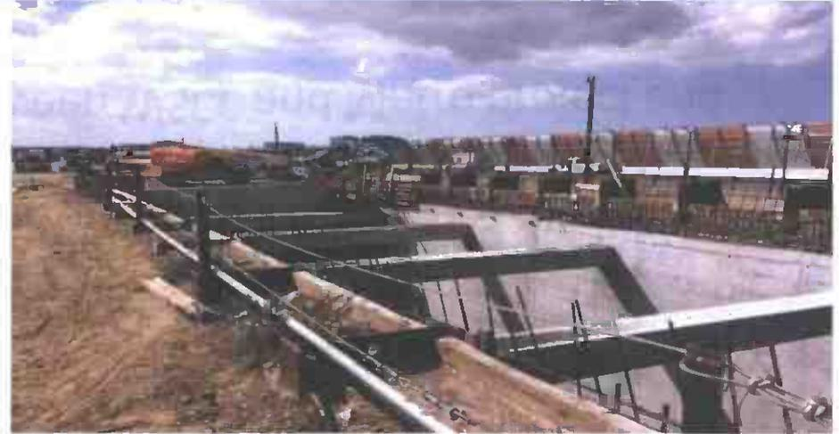
**UG#1– Concrete barrier formwork installation on the west U-wall
