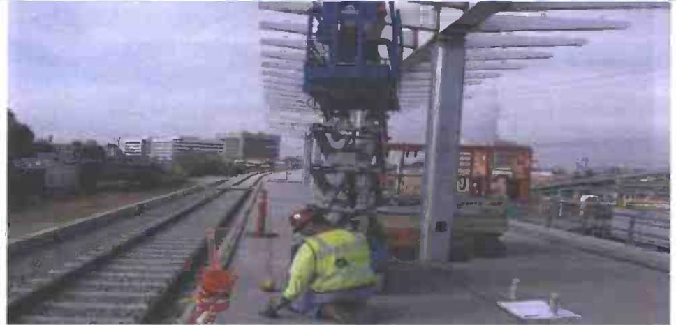
LA BREA AT GRADE STATION – Completed canopy outrigger welding and electrical and plumbing installations
