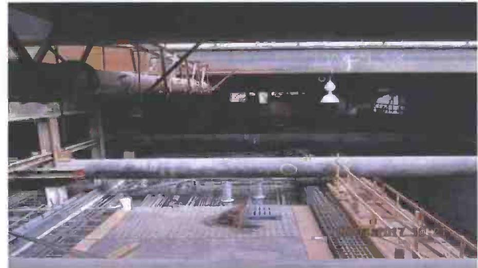
**EXPOSITION/CRENSHAW STATION – Installing rebar for roof slab phase 1**
