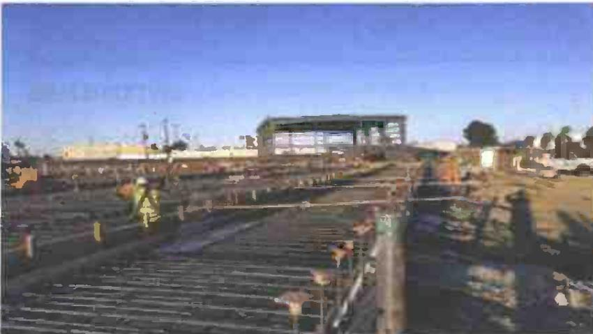
**Placing reinforcement for car wash slab**
