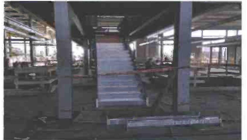
**Installing stairs to service platform**
