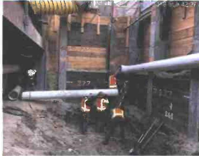
Storm drain bypass at south access shaft
