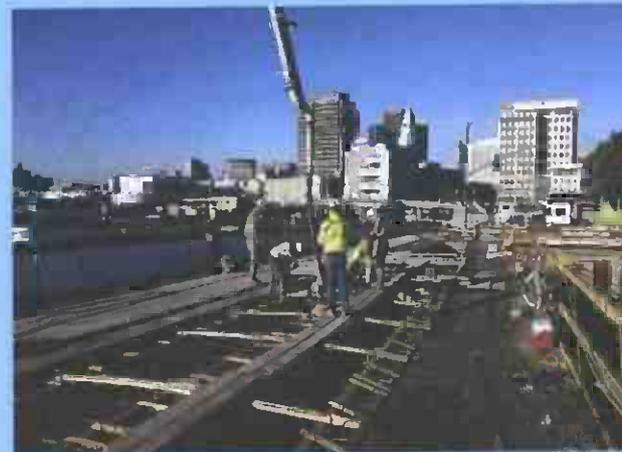
Pouring Stems and Soffit
