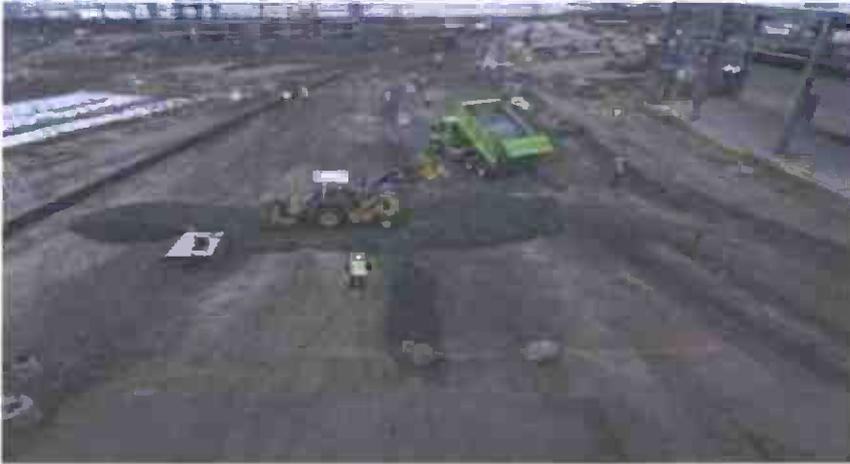
**Dumping ballast at underdrains**
