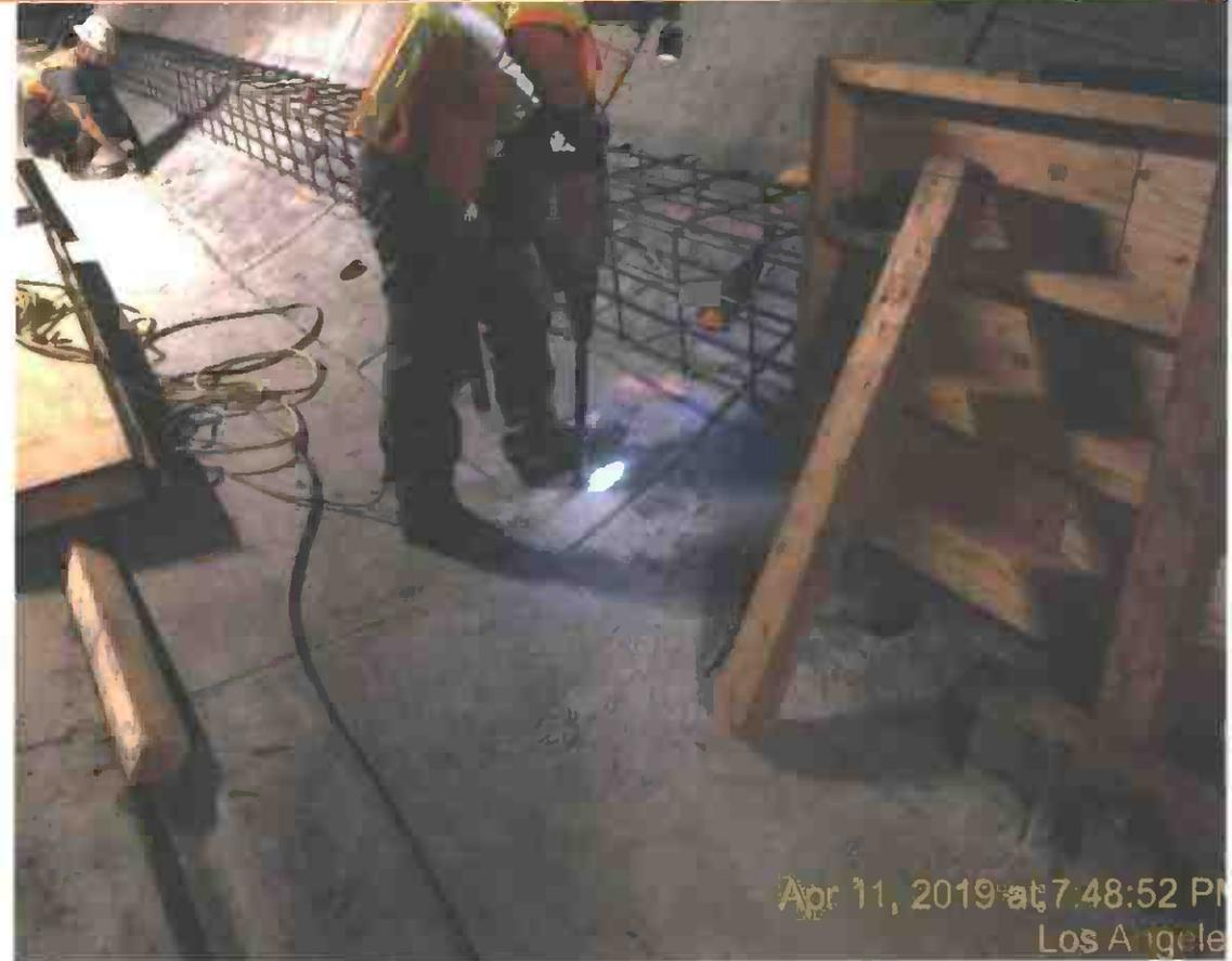
Floating Slab Track curb formwork installation
