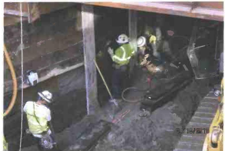
Installation of TBM Launch Box Lagging
