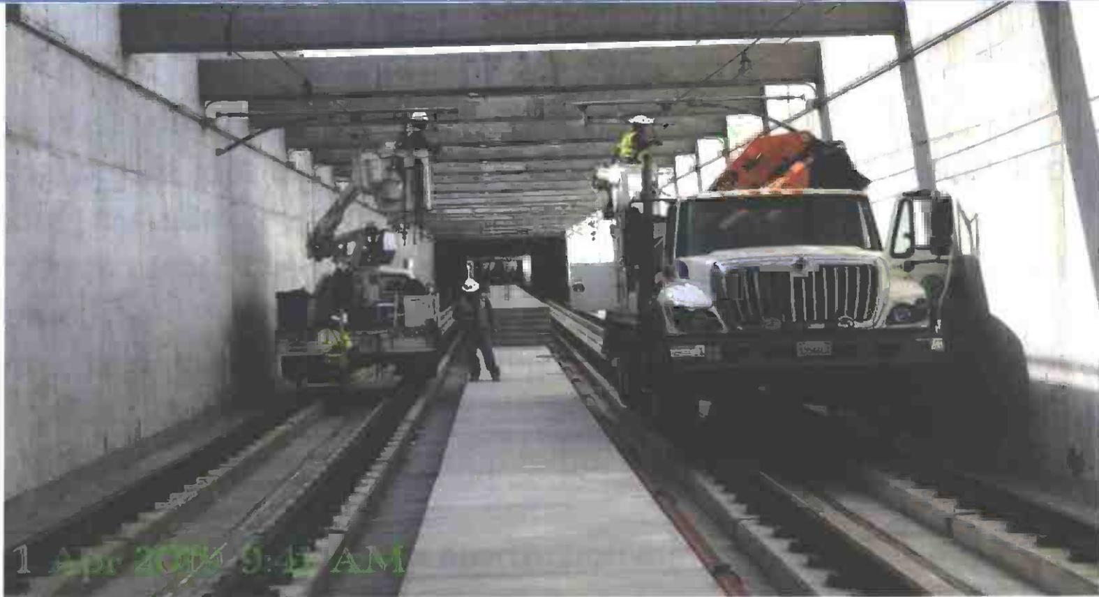
Systems subcontractor LKC continues work on overhead contact system at Underground Tunnel #1
