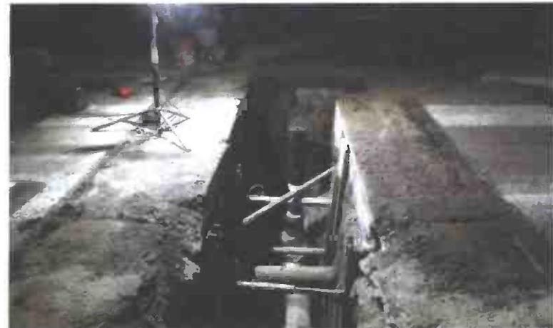
Gate Valve Steel Lateral Installation
