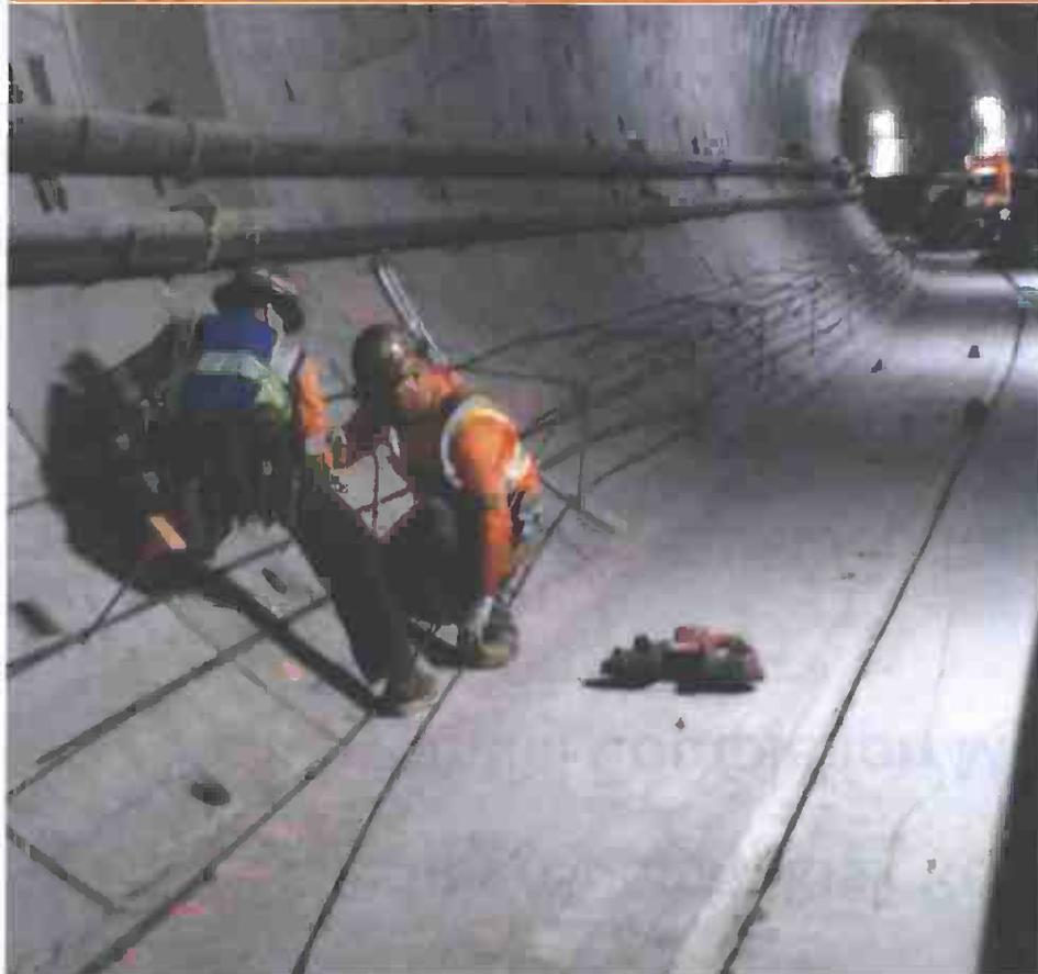
Installing Floating Slab Track curb rebar
