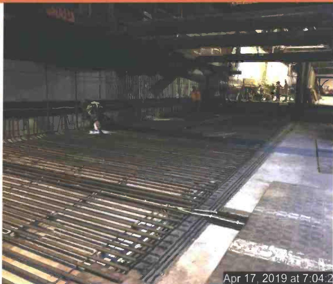
Bottom mat rebar installation at FCC-7 and FCC-8
