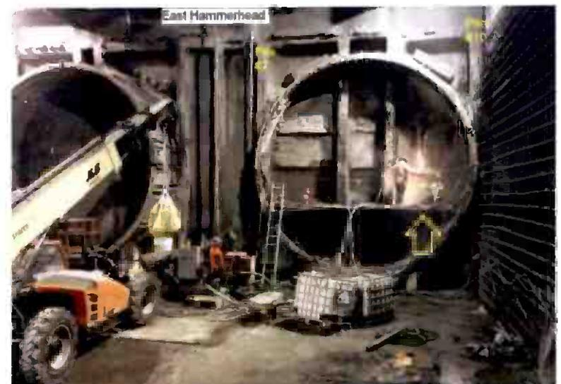
Installing Shotcrete at Tunnel Eye
