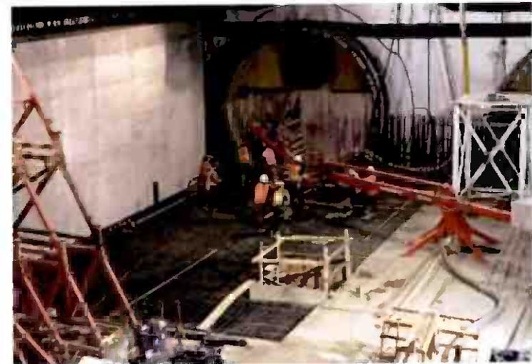
Infill Slab Concrete Placement at North Wall (Platform Level)
