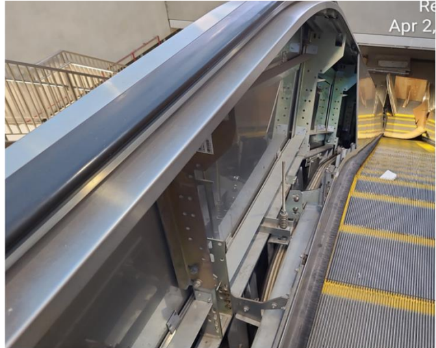
Stainless steel cladding installation PE1 escalator at Little Tokyo/Arts District Station
