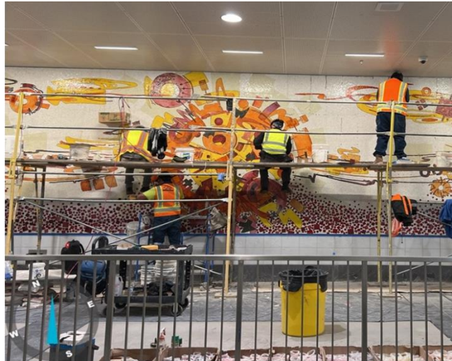
Mosaic art glass installation touch ups at Historic Broadway Station
