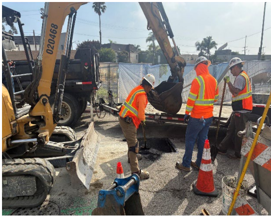
San Vicente Street Restoration
