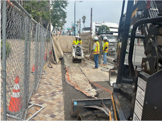
Wilshire Blvd. Trenching for Conduit Installation
