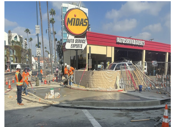
Wilshire Blvd. and N Le Doux Road Curb Ramp Construction
