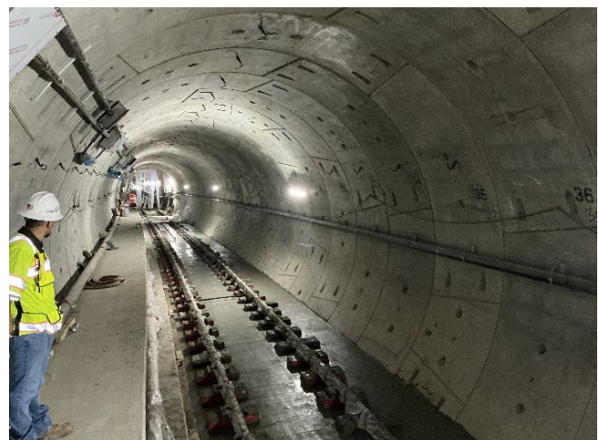
BR R5 Completed Infill Placement
