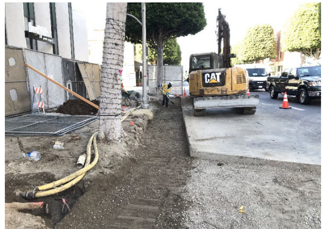
BDS Bus Pad Construction
