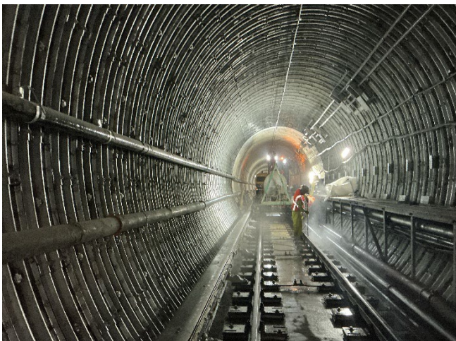
Pressure Washing at Seismic Zone
