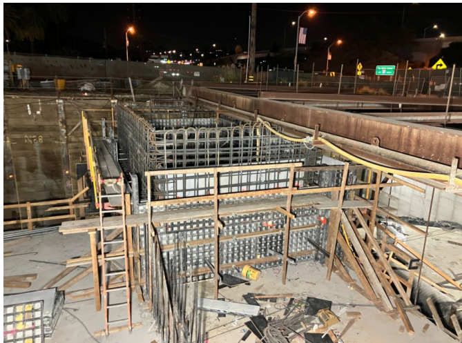
Westwood/VA Hospital Station: Roof Appendage Walls Construction Facing North
