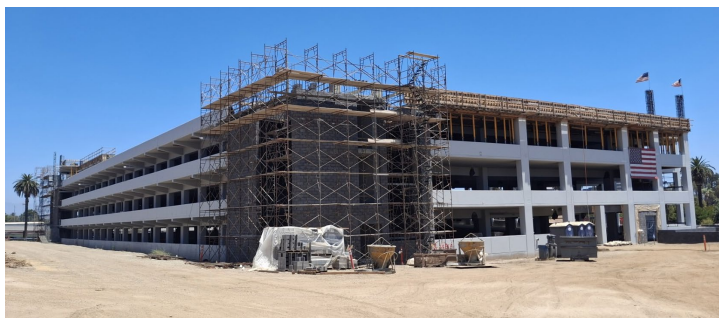
Parking Structure: VA Parking Structure, Facing Southeast
