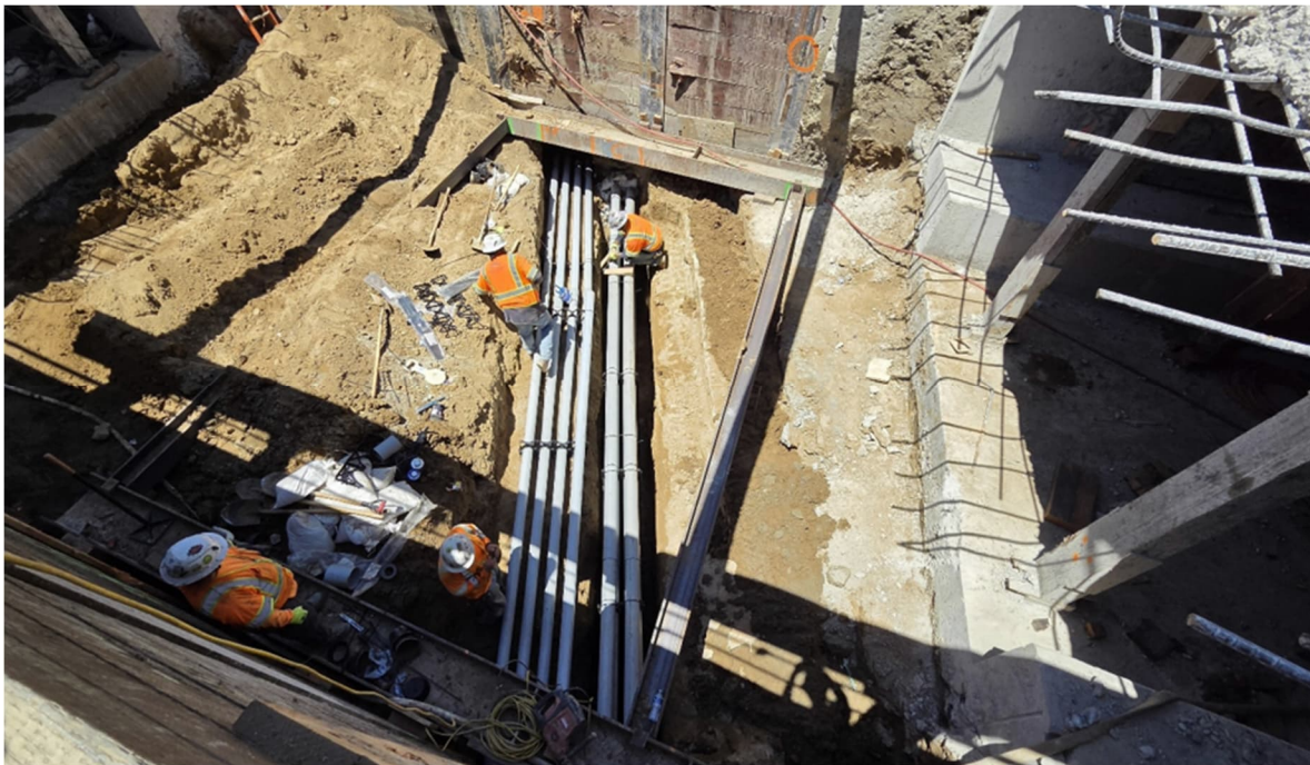
SFTC crew installing conduits for Metro Systems ductbank Segment A2 under Pacoima Wash Culvert, Van Nuys Blvd
