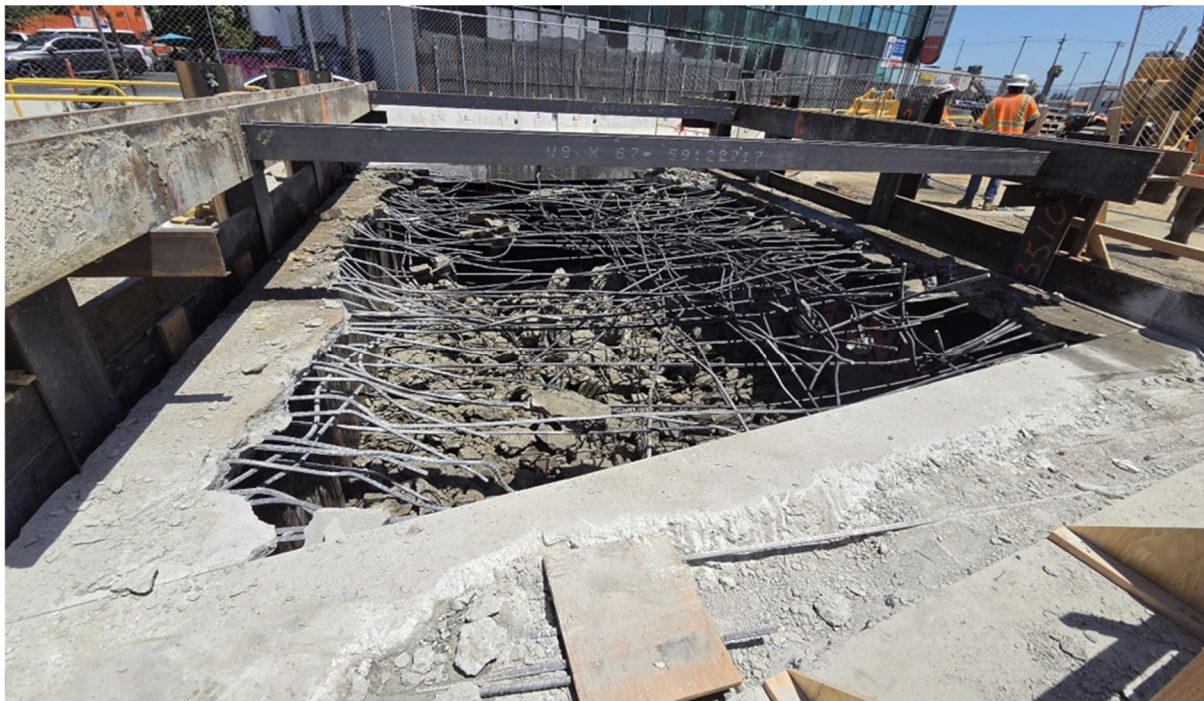
Support of excavation installed and Pacoima Wash Culvert Roof (street level) demolition Pacoima Wash Culvert, Van Nuys Blvd, South of Covello St
