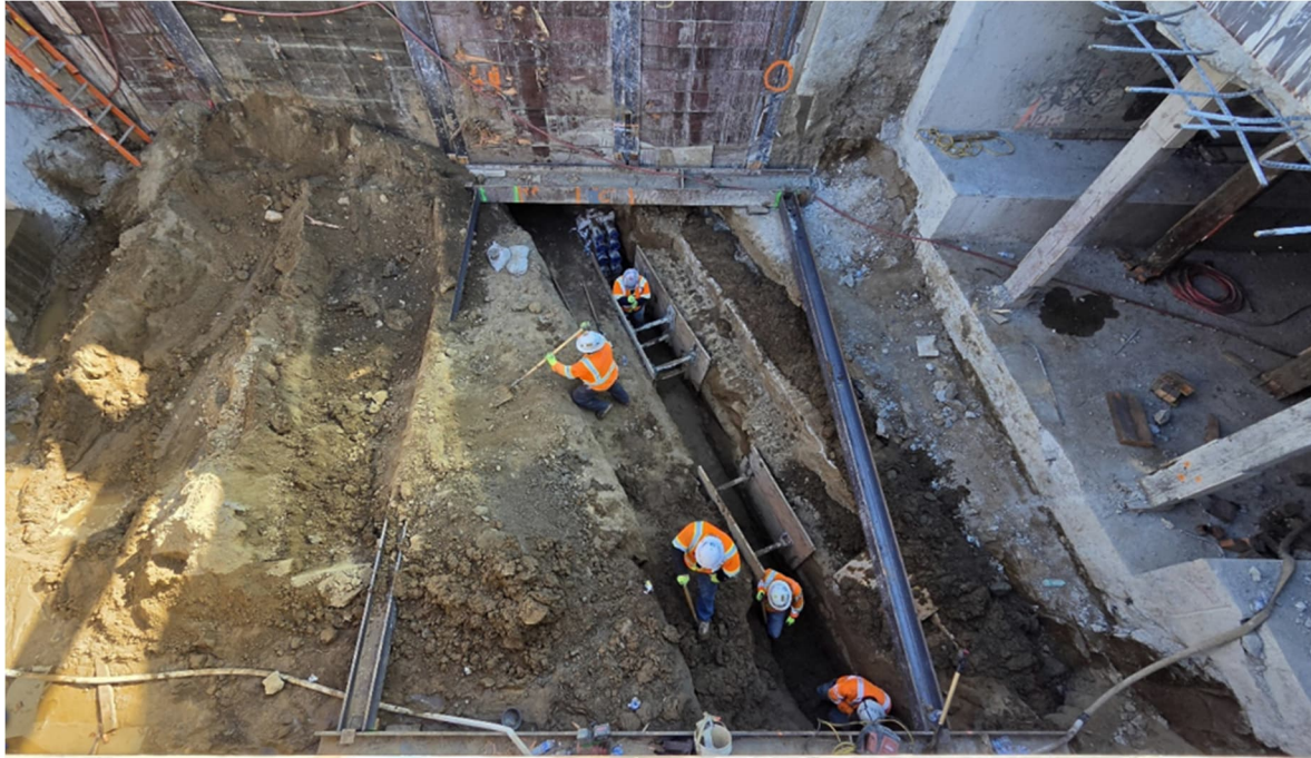
SFTC excavating and shoring trench for Metro Systems ductbank Segment A2 under Pacoima Wash Culvert, Van Nuys Blvd
