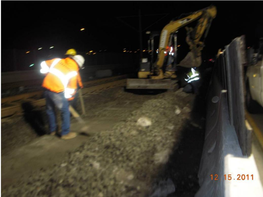
Looking at trench excavation inside railroad Right of Way, working behind k-rail. Preparing the location for shoring to protect track work during pile excavation.
