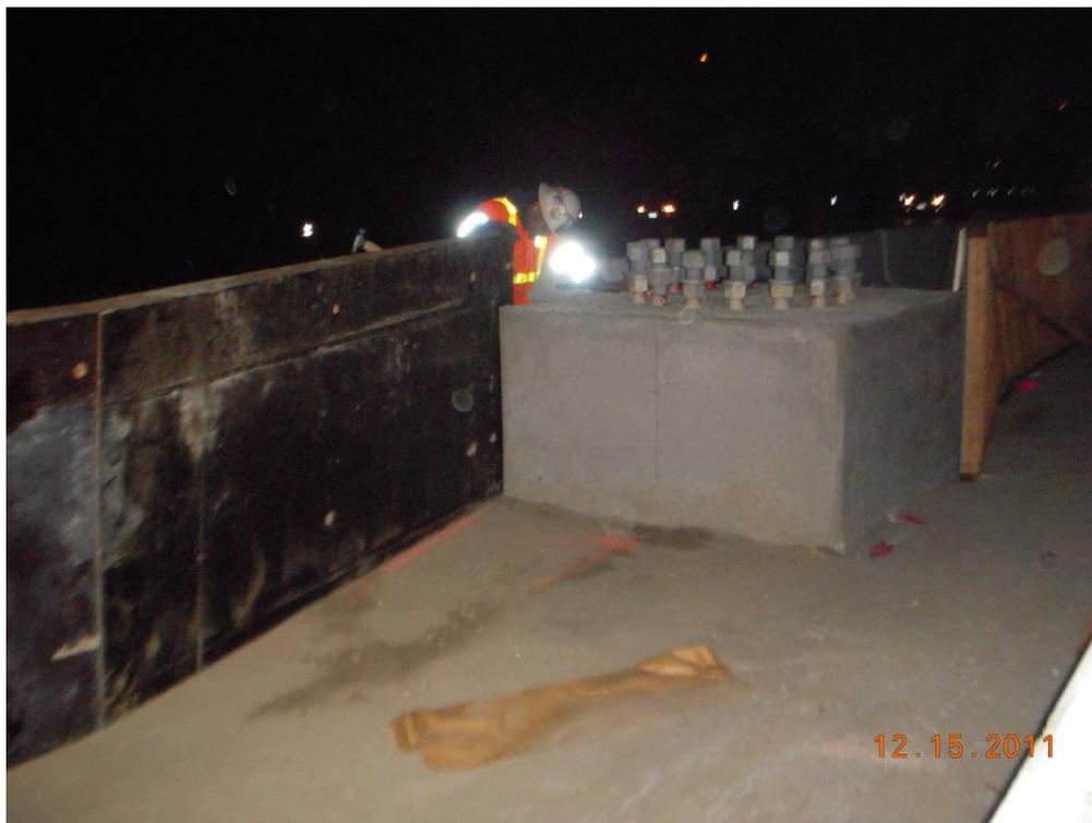
Looking at the inside of forming for a new medium pour next to a new sign foundation.
