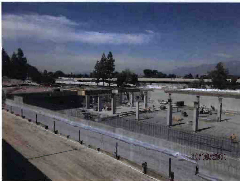
Site photo looking west.
