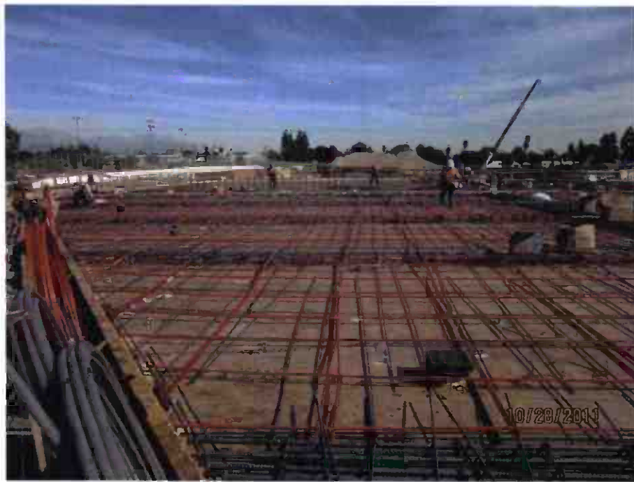
Deck No 1 rebar and PT tendons.
