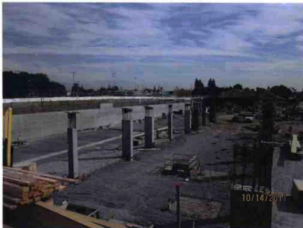
North ramp wall from elevated decking.
