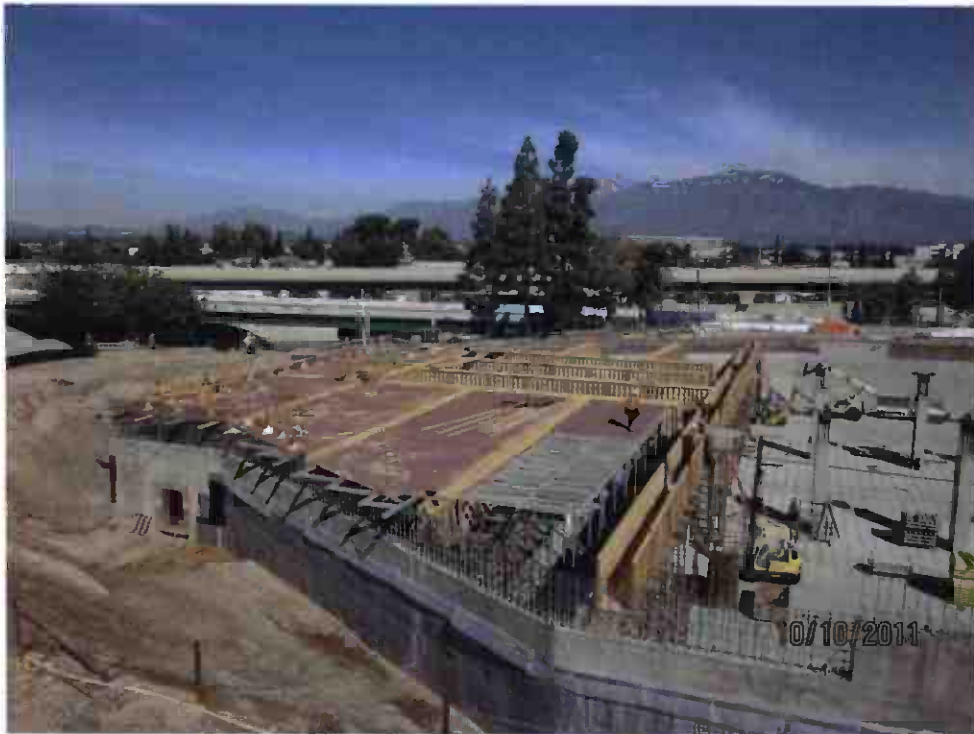
West end elevated decking.
