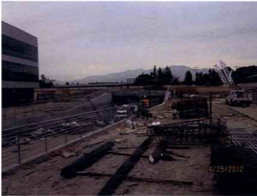
Installing handrails above ramp.
