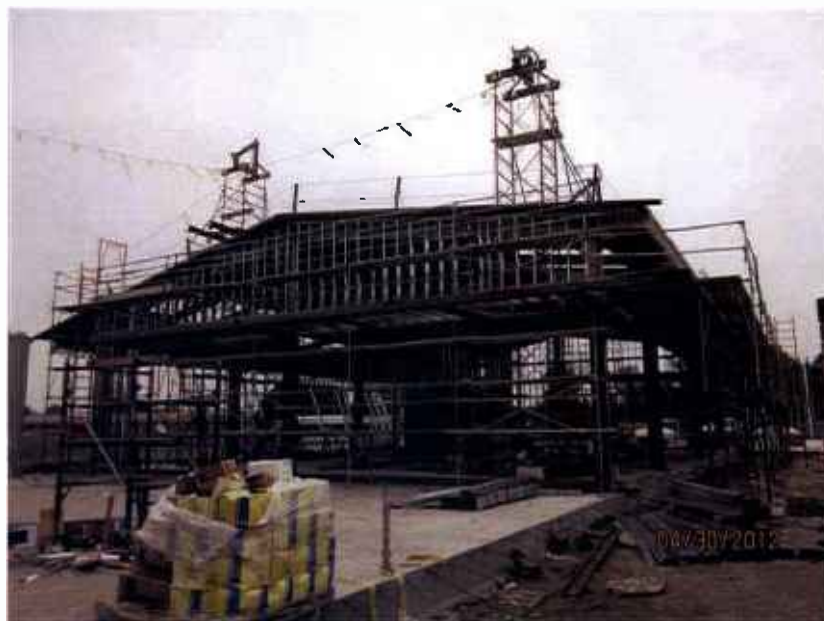
Site steel erection.
