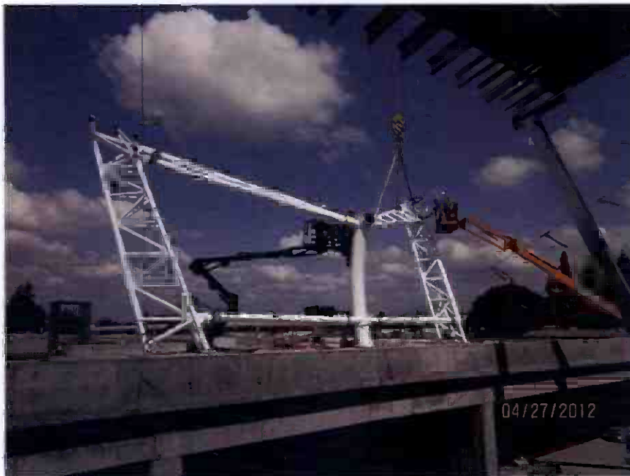
Canopy steel erection.
