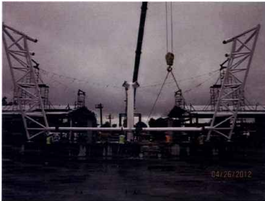
Setting canopy support steel.
