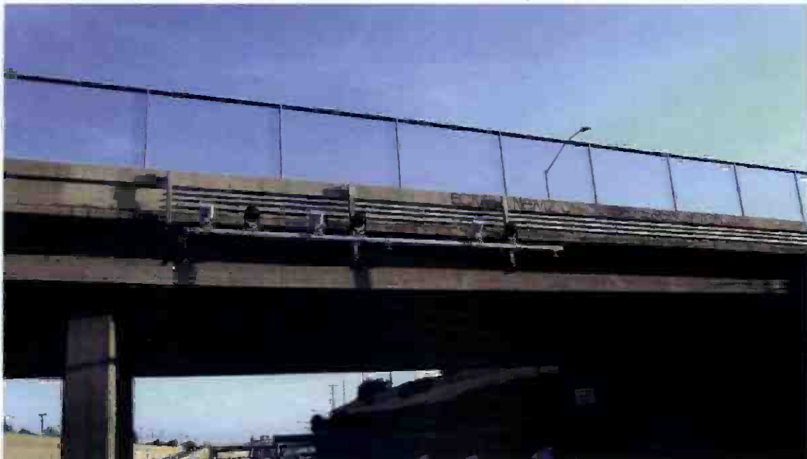
DSC 1134 new camera's attached to a bridge on I-110
