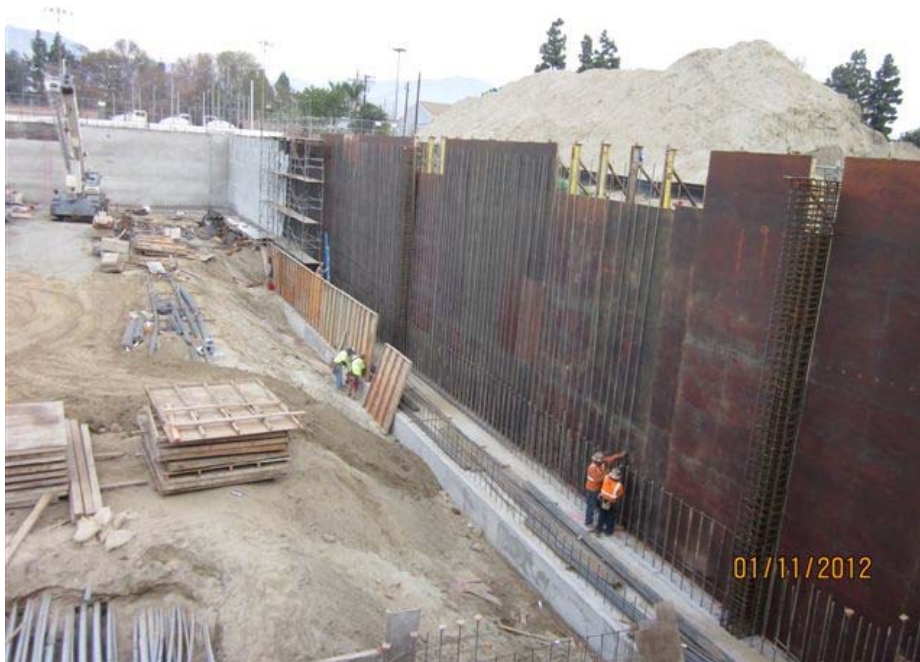
Setting HVAC wall forms.
