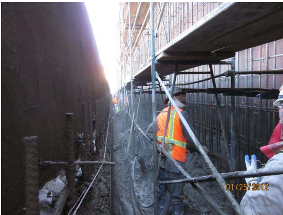
Shooting shotcrete on line #26.
