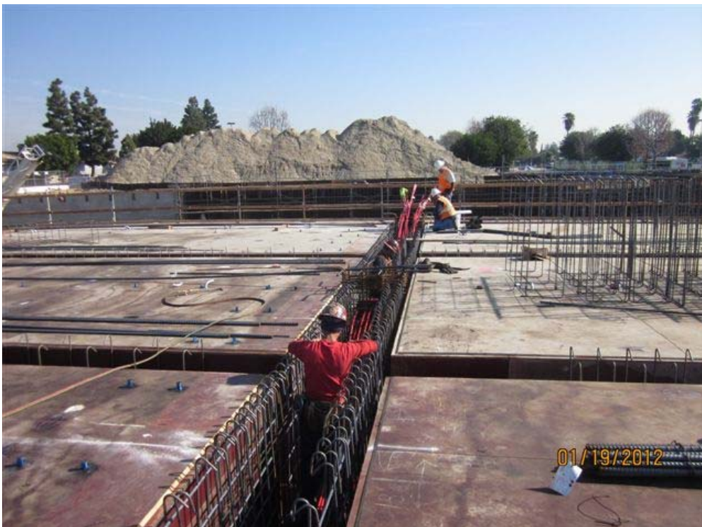
Building rebar beams on Deck #7.
