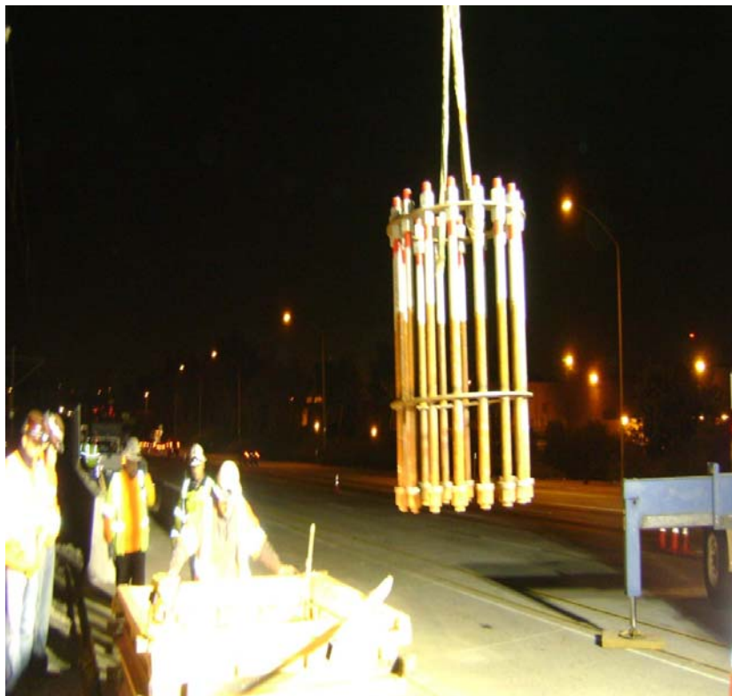
Base support bolts being placed.
