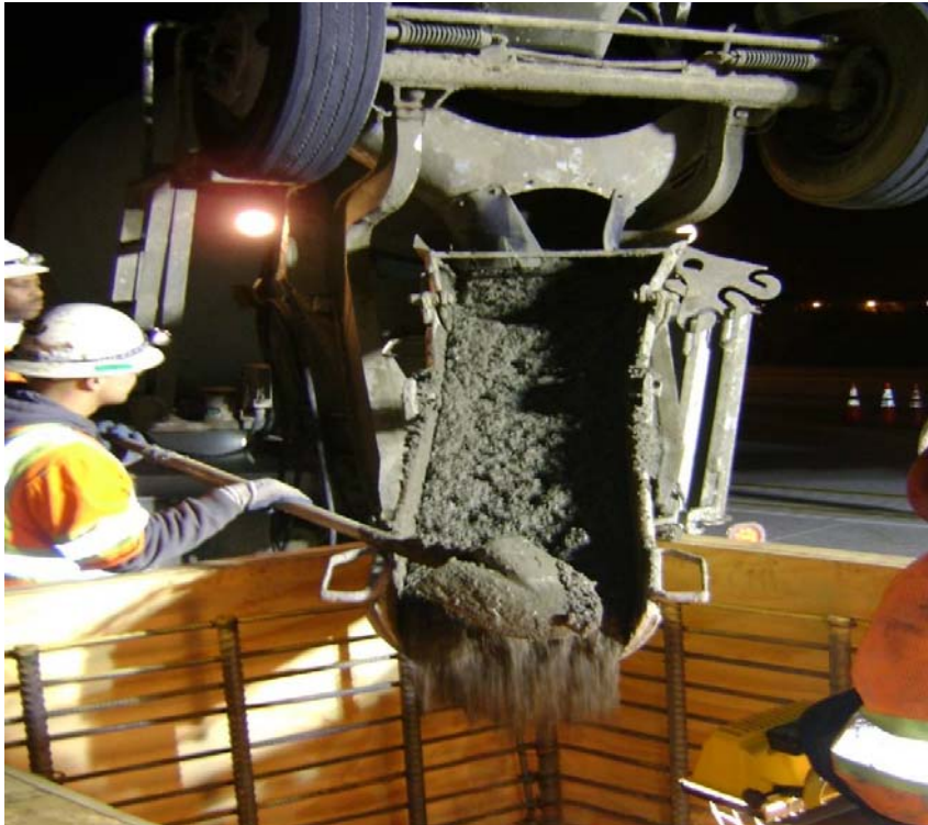
Pouring of foundation Pile 560.
