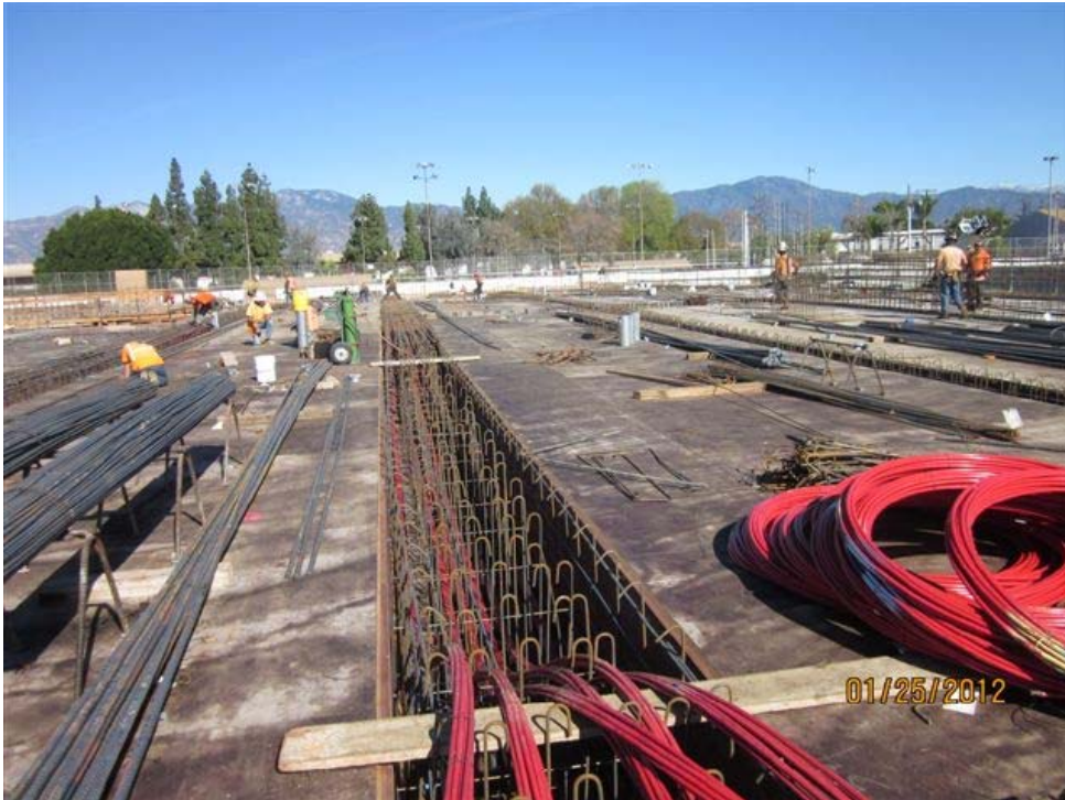
Deck #7 rebar beam.
