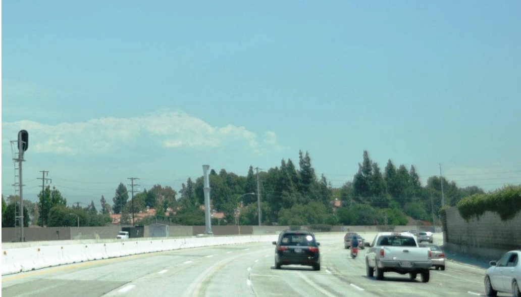
Median work at east end of I-10 Freeway.
