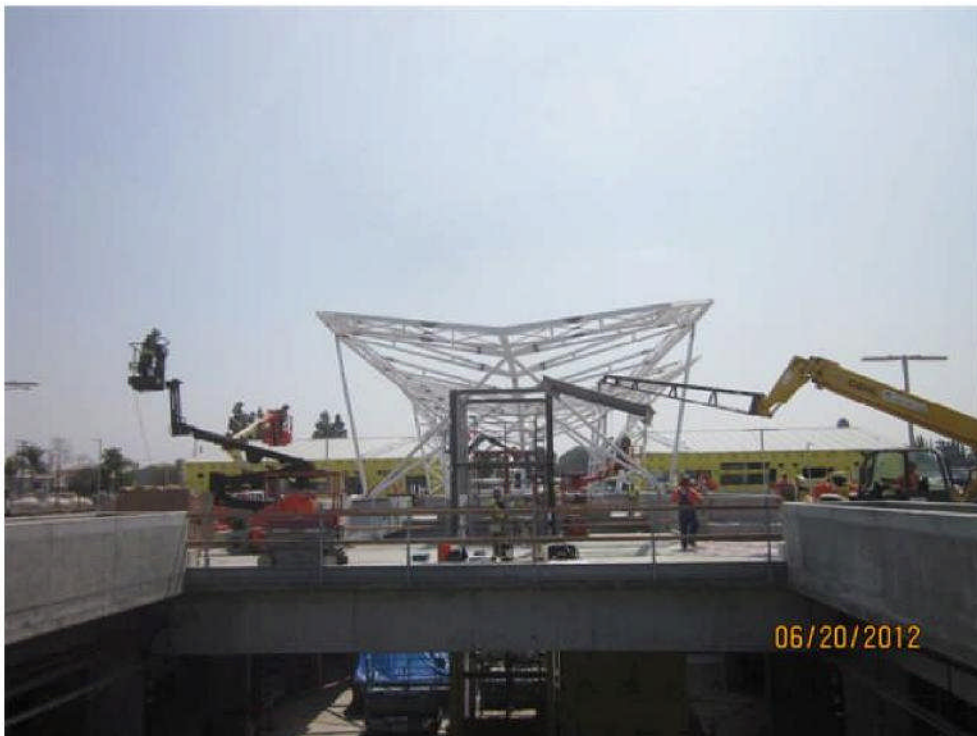
Site photo looking east.
