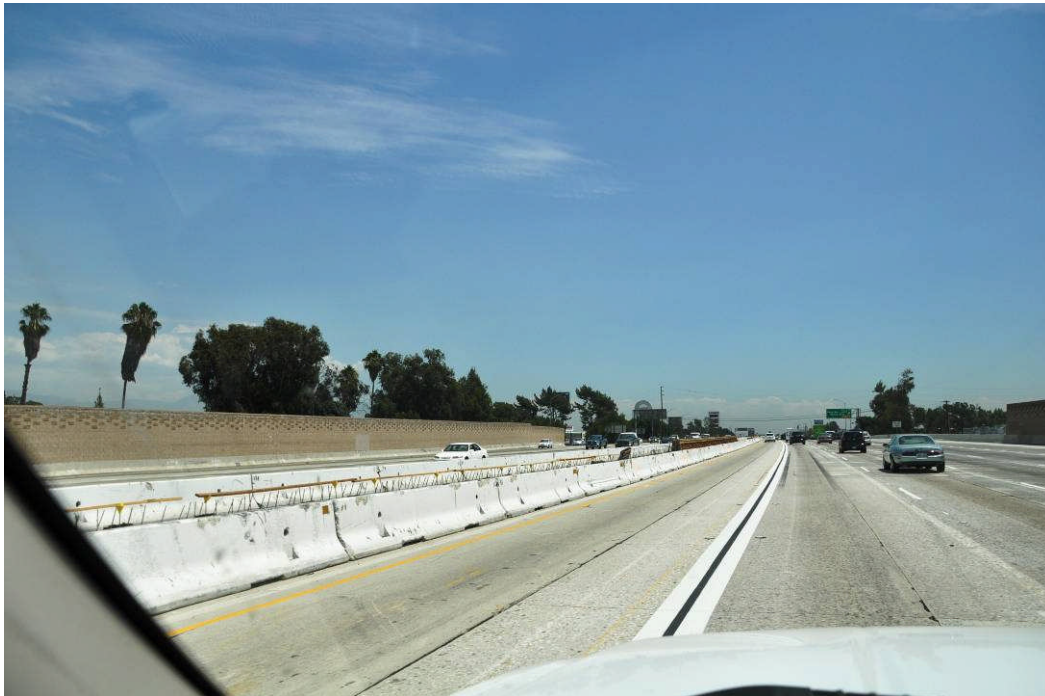
Median work at east end of I-10 Freeway.
