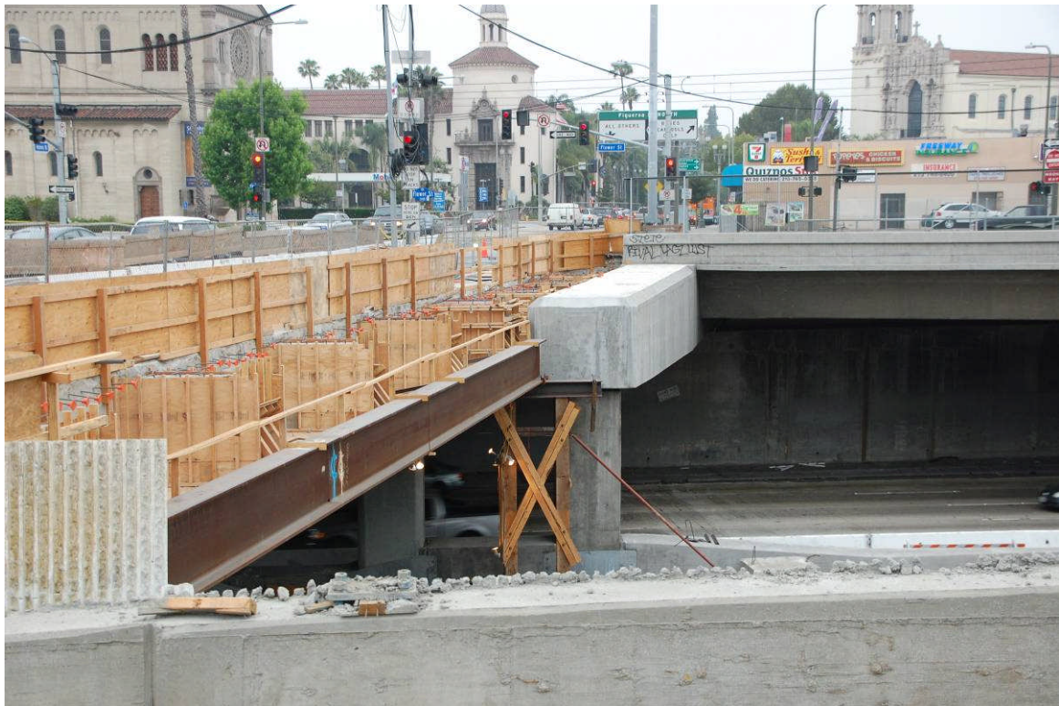
FW over NB traffic facing.
