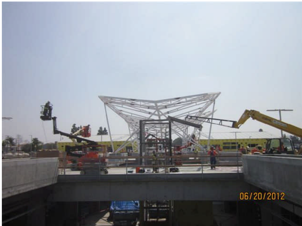
Setting elevator hoistway extension.
