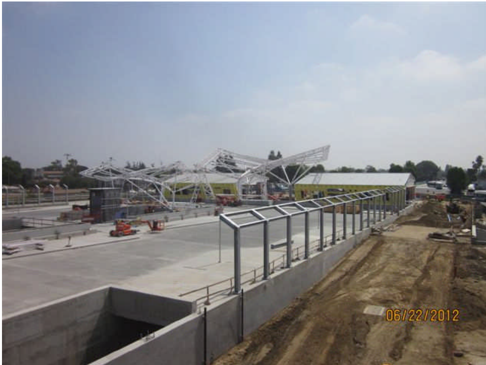
Site photo o looking east.
