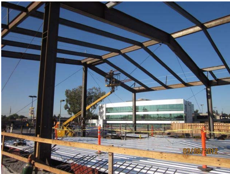
Installing roof bracing on retail building.
