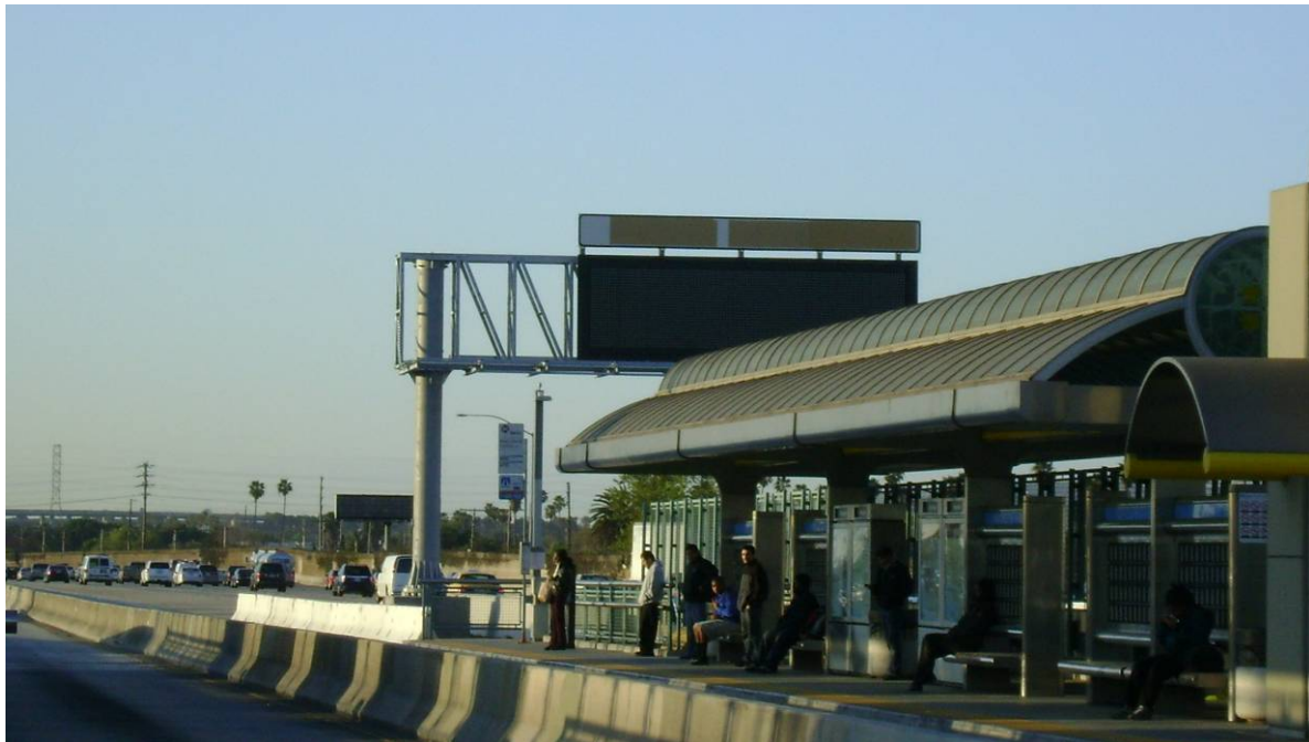
Sign 290 facing SB direction along I-110.
