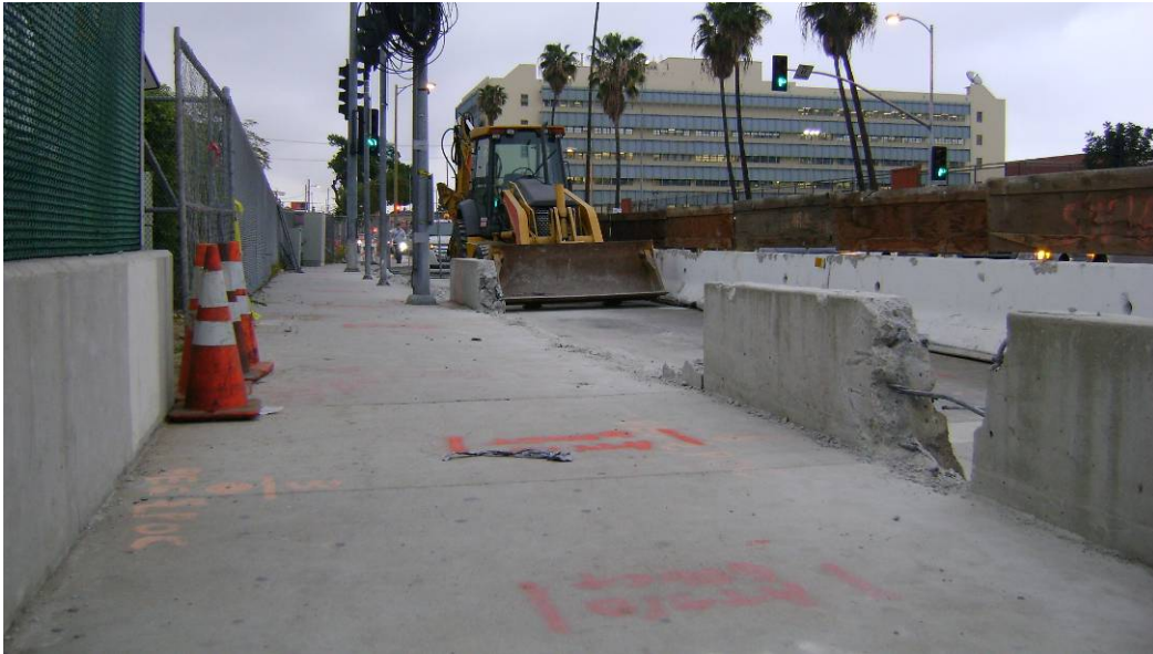
Facing east on Adams Blvd. barrier removal.
