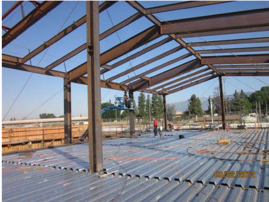
Welding steel framing on transit building.
