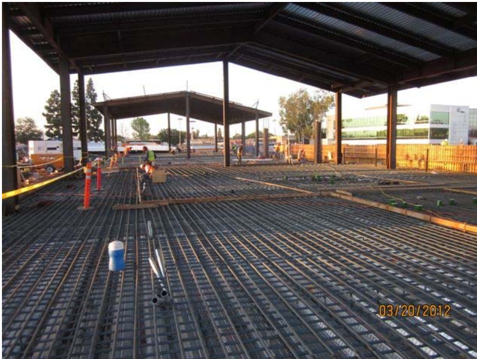
Looking south in buildings.
