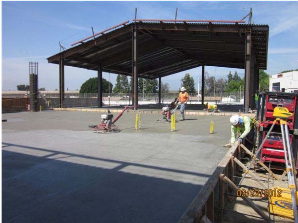
Concrete finish on building slab.
