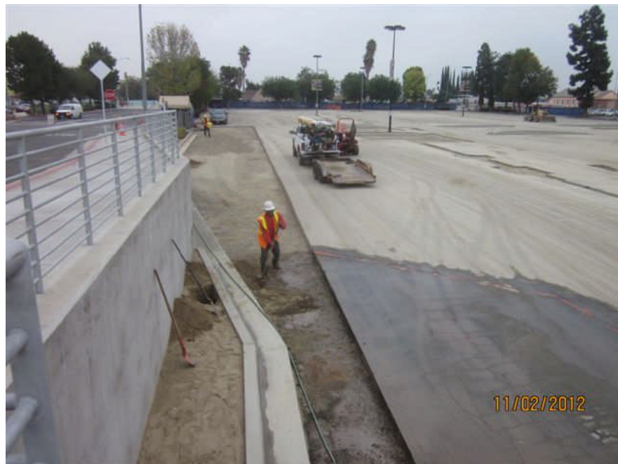
Trenching in irrigation lines in Lot B.
