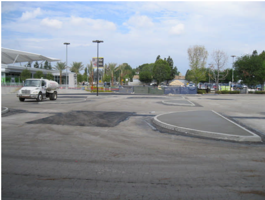
Island infill with concrete.
