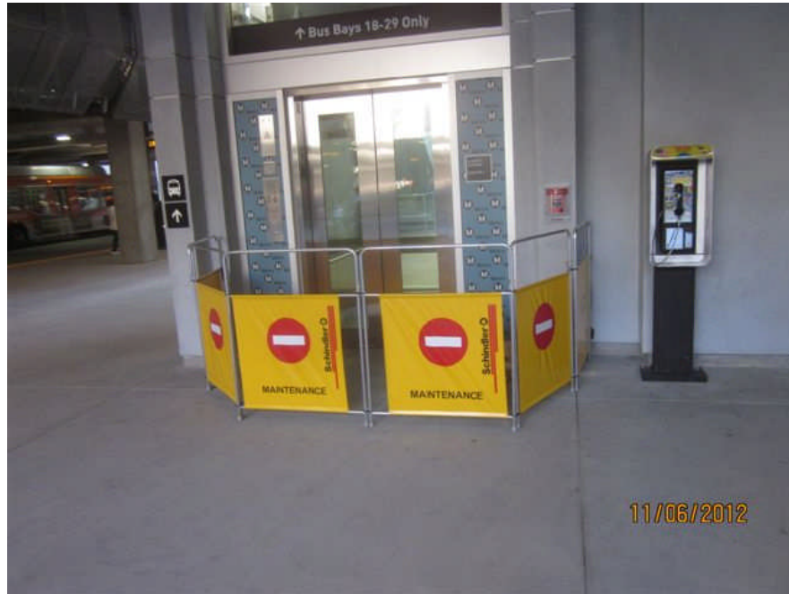
Punchlist work taking place on elevator no. 2.
