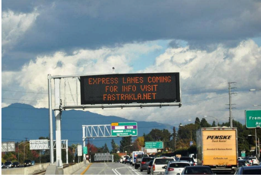
DMS sign close to Fremont Ave on I-10 freeway.
