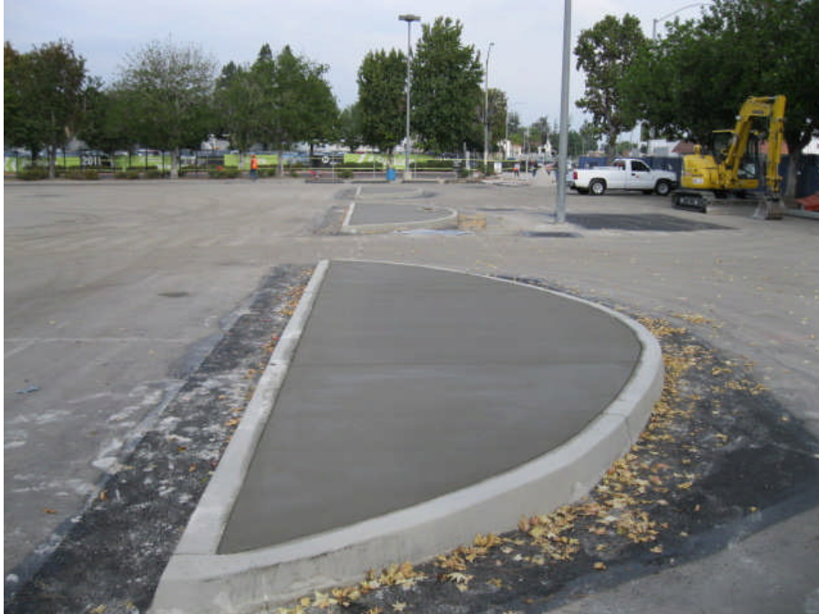
Concrete placement Lot B islands.
