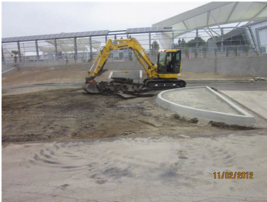
AC removal in Lot B.
