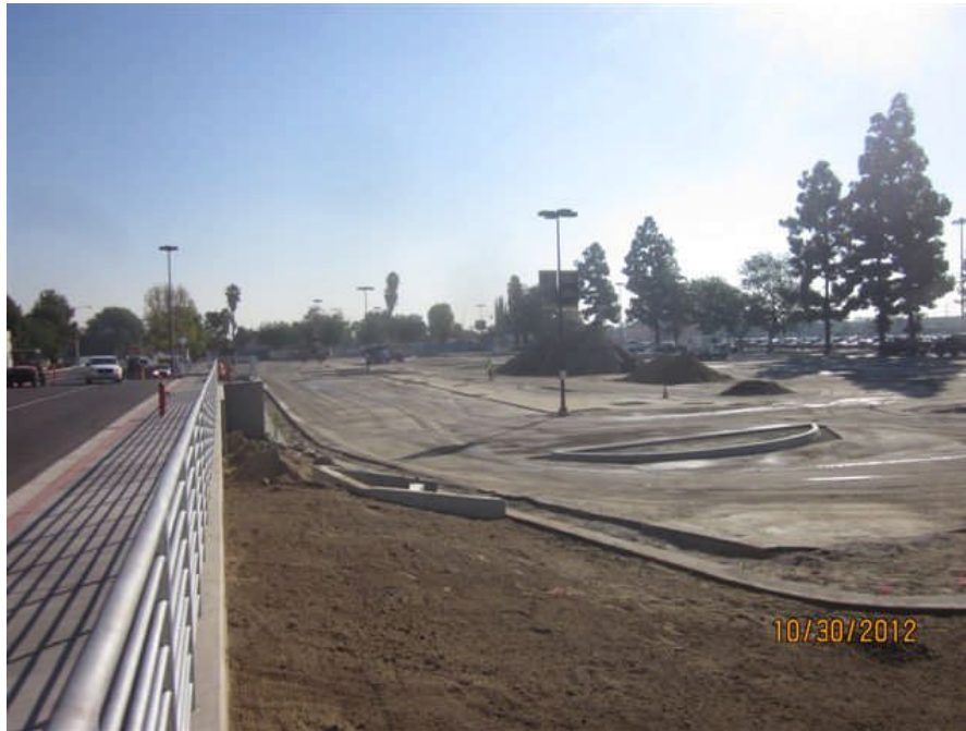
Curb and gutter in place.
