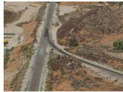
Vista Canyon Station – Before
