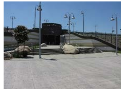
Vista Canyon Station – After
