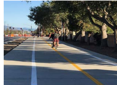
Hollister Avenue Bike Path – After
