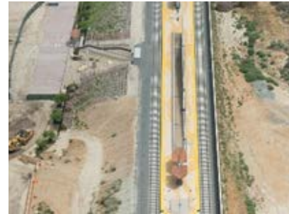
Vista Canyon Station – After
